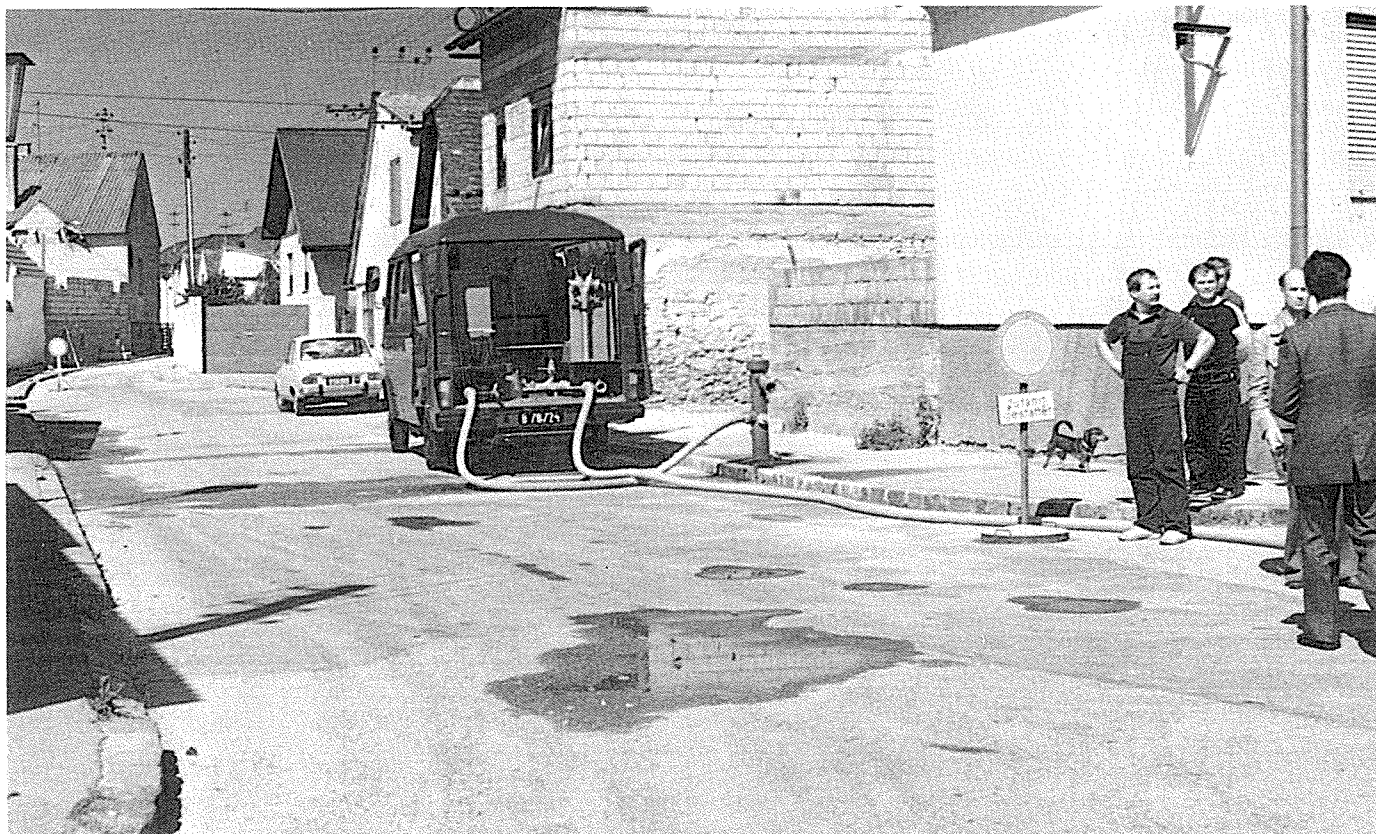
A mobile water control unit used in Europe for water loss analysis in municipal water supply systems. A similar unit will be used in the local research project on water loss analysis.
