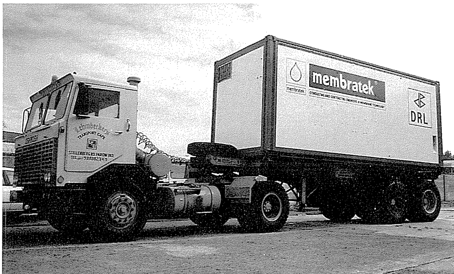
The mobile pilot-scale sea-water desalination plant of Membrattek and De Beers research laboratory.
