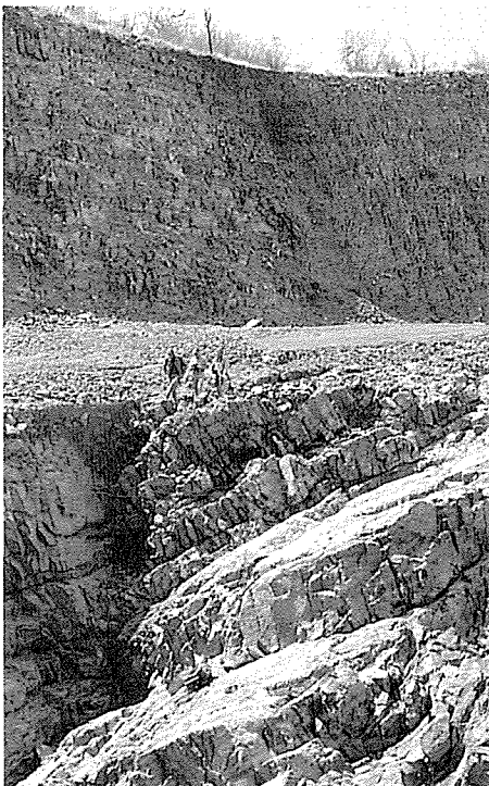
Hans Strydom Dam: Erosion along the fault zone, in the spillway channel.
