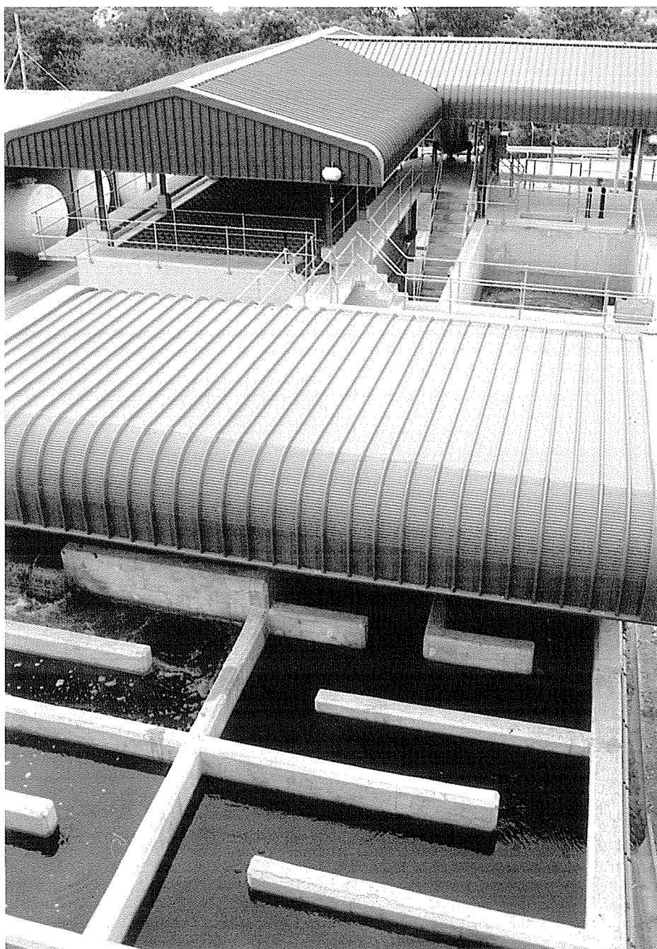
Flotation plant for the treatment of eutrophic water to drinking water.
