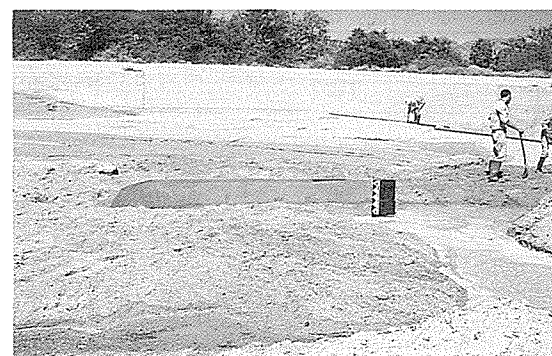
Olifants River at Barandas: These photos show the problems experienced at the gauging weir as a result of high sediment levels in the pool. The pool must be cleaned regularly to enable meaningful measurements to be made at the gauging weir
