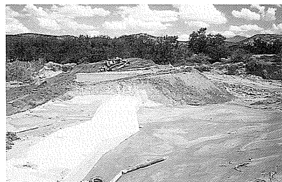
Olifants River at Barandas: These photos show the problems experienced at the gauging weir as a result of high sediment levels in the pool. The pool must be cleaned regularly to enable meaningful measurements to be made at the gauging weir
