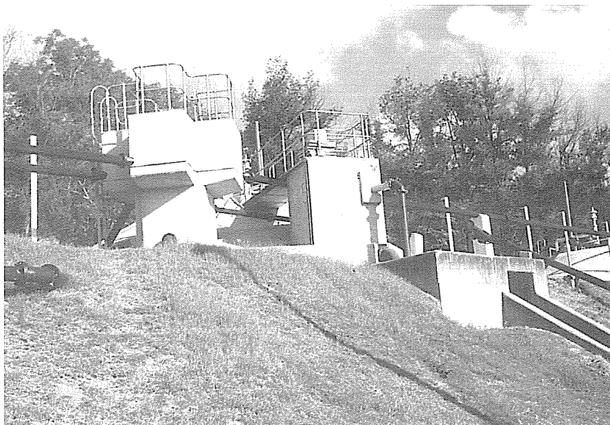
General view of the earth-covered digester at Umbilo Sewage Purification Works in which concentrated dye effluent is being treated.
