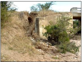
**Figure 3-27:** Channelling of stormwater from the road or bridge surface into the river channel may aggravate the effects of local scour behind abutments shown in the previous figure, NB0960, Limpopo Province.
