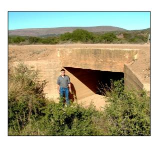
Figure 3-12: Constriction of the flow at this culvert near Riebeeck East, northwest of Grahamstown, Eastern Cape, has led to high velocity water exiting the downstream end. The riverbed has been severely scoured for a long distance downstream.
