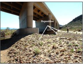
**Figure 3-25:** Deposition downstream of one of the bridge piers shown in Figure 3-24
