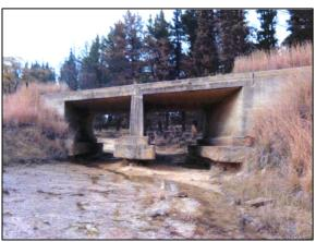
**Figure 3-17:** The above bridge is in a critical state as constriction scour has eroded the riverbed under and downstream of the structure, exposing the foundations completely. (Photo: Free State Department of Transport)
