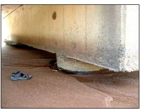
**Figure 3-5:** Evidence of local scour at the piles in the sandy riverbed.
