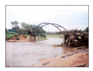
**Figure 3-32:** The approach embankments of a bridge in Dainfern Golf Course, Gauteng, were washed away during 2000. (Photo: Arup, 2000)
