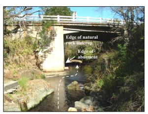
**Figure 3-31:** Poor alignment of this bridge in Swellendam, Western Cape, has led to local scour upstream of the abutment.
