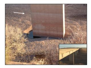
**Figure 3-22:** Local scour holes are not often visible as they may be under water or filled with sediment after floods. The local scour hole at a pier of this bridge near the Gariep Dam is clearly visible (bridge inset).
