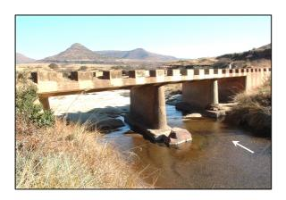
**Figure 3-20:** A local scour hole has developed at the closer pier in the soft riverbed rock at this bridge south of Aliwal North, Eastern Cape
