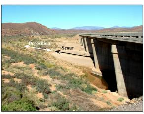
Figure 3-19: Bridge B5007, between Ladismith and Riversdale over the Touws River, in the Western Cape demonstrates the action of constriction on a large scale. Scour occurred under and immediately downstream of the bridge. Deposition of the sediment is evident further downstream where the river channel is more vegetated.
