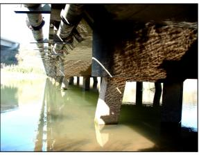
**Figure 3-7:** The piles of this bridge near the Mzimkulu river mouth have been exposed to a significant depth.
