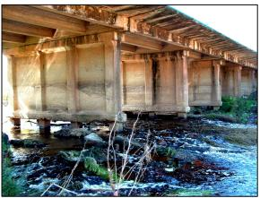
**Figure 3-9:** The Palmiet River in the main street of Grabouw, Western Cape, no longer flows parallel to the bridge piers. This may have initiated scouring under the bridge and exposure of the piles.
