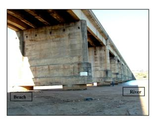
**Figure 3-8:** Caissons below the N2 Bridge at Port Shepstone are exposed.
