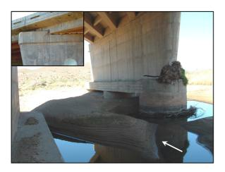
**Figure 3-24:** Local scour holes at the Touws River Bridge between Ladismith and Riversdale, Western Cape. Some differential movement between the piers and bridge deck has occurred (inset).
