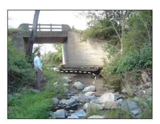
**Figure 3-28:** The river approaches the abutment rather than the opening of culvert NB241 in Limpopo Province.
