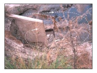
**Figure 3-26:** Local scour downstream of the bridge abutment erodes the approach embankment behind the wing-wall of bridge B0896, Free State. (Photo: Free State Department of Transport)
