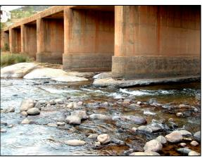
**Figure 3-11:** Although repair of the scouring under this bridge is not urgent, mining of river sand downstream of structures can initiate head-ward erosion which could undermine the foundations.
