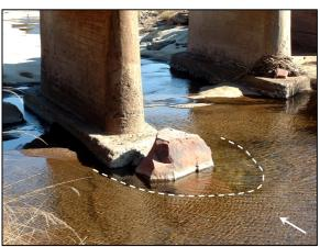
**Figure 3-21:** Detail of the local scour hole at pier shown in Figure 3-20.
