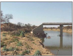
**Figure 3-33:** Outflanking of the bridge abutments and scour of the riverbed has exposed the piles anchoring the abutment at this bridge in Limpopo Province. (Photo: Leporogo Specialist Engineers)
