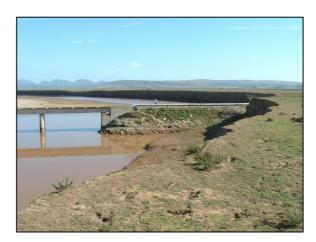
**Figure 3-34:** Bend scour on this meander of the Gouritz River near Gouritsmond, Western Cape, is threatening the bridge abutment and approach fill on the far side.
