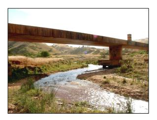
**Figure 3-2:** General scour, occurring as the river naturally erodes downwards, has exposed the piles at some pier footings at bridge ZB1103 near Dalton, KwaZulu-Natal.
