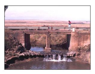
**Figure 3-16:** Scour downstream of B1972 in the Free State (Photo: Free State Department of Transport)
