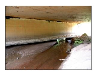
**Figure 3-4:** Water flows under the bridge piers as a general lowering of the bed has occurred at B2763 near Glendale, KwaZulu-Natal. This bridge is also subject to excessive sedimentation at times.
