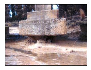
**Figure 3-18:** The bridge piers are not founded on piles or caissons and are resting only on small quantities of directly-compressed material. (Photo: Free State Department of Transport)
