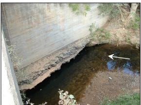
**Figure 3-29:** The abutment has been undercut laterally by about 1.5m.
