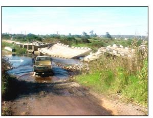
**Figure 3-23:** This bridge in the town of Heidelberg, Western Cape, failed as the foundations were undermined. The fact that piers on the *upstream* side failed suggests that local scour was responsible.
