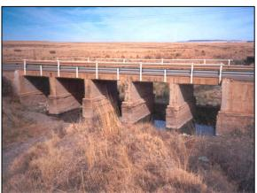
**Figure 3-15:** Scour of the riverbed immediately under the bridge openings may indicate constriction scour. Many bridges such as this have puddles of stagnant water under the structure where scour took place during floods. (Photo: Free State Department of Transport)
