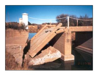
**Figure 3-30:** The above abutment and one bridge span failed as the abutment was undercut. (Photo: Free State Department of Transport)
