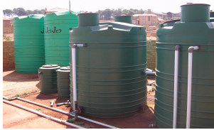
Submerged bio-contactor
