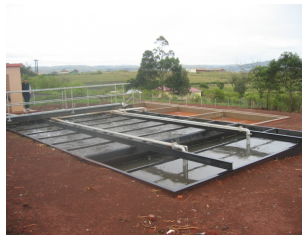
Activated sludge package plant
