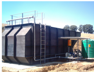
Activated sludge package plant
