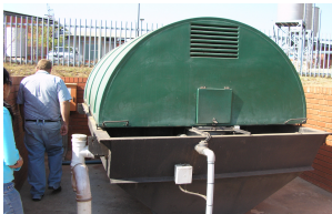
Rotating bio-contactactor
