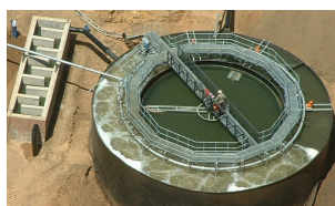
Extended aeration installation
