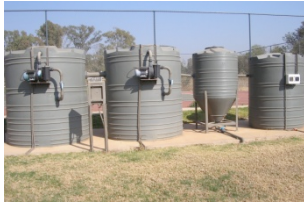
Submerged bio-contactor installation
