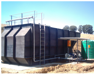
Example of a package plant installation
