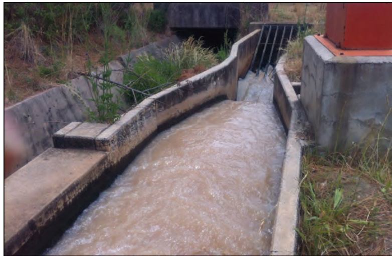
Figure 7-15: The inlet to a siphon on the Sand River canal system (DWA, 2013)
