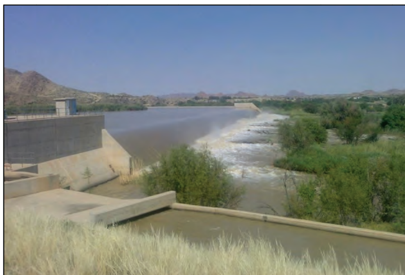
Figure 7-4: Typical measuring structure/weir
