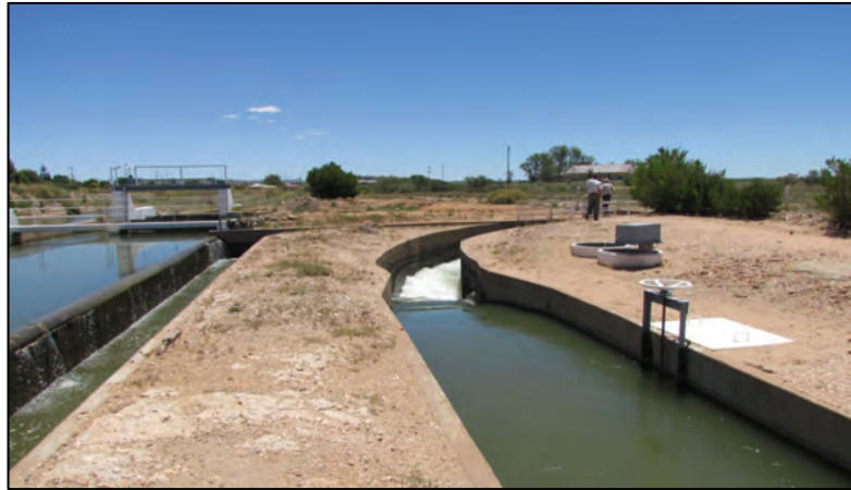
Figure 7-9: Diversion structure in the Boegoeberg Irrigation Scheme (DWA, 2013)
