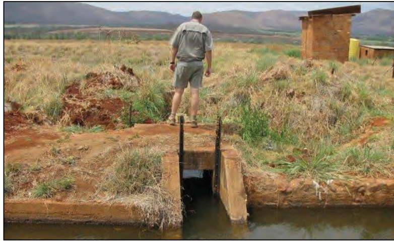
Figure 7-10: Sluice with almost no hydropower potential (DWA, 2013)
