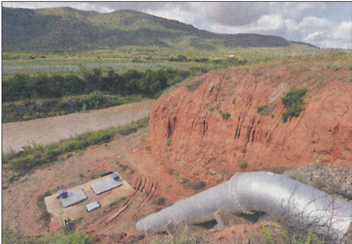
Figure 8-4: Penstock to Ossberger turbine (Botha, 2013)
