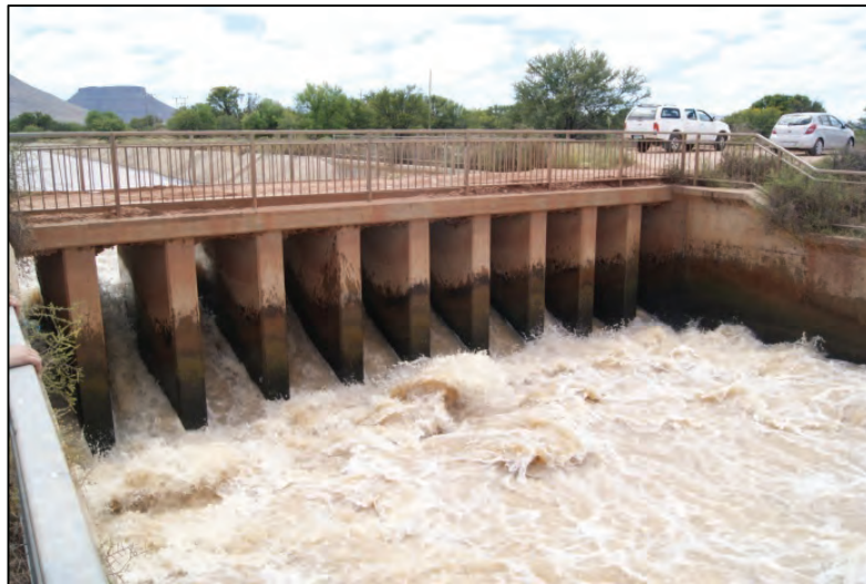
Figure 7-11: Energy dissipating structure (at bridge) in Teebus canal (Orange-Fish Transfer Scheme)
