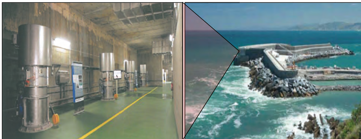
Figure 7-26: 300 kW Oscillating water column Mutriku wave power plant in Spain (Voith, 2011)
