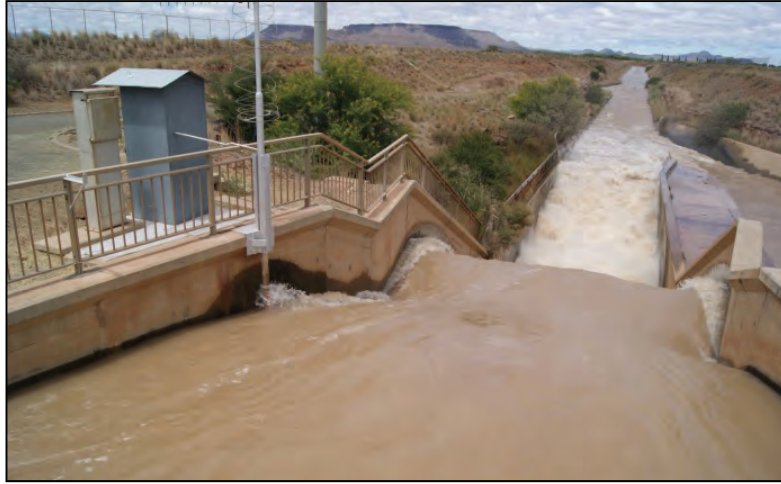
Figure 7-12: Flow gauging telemetry system at the Teebus canal (Orange-Fish Transfer Scheme)
