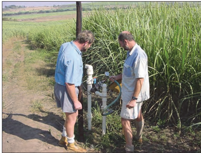
Figure 15 Pressure being checked at the irrigation block inlet (Koegelenberg & Breedts, 2003)
