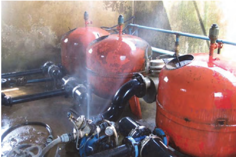
Figure 20 Water leaks increase flow requirements and reduce efficiency (Horn, 2014)
