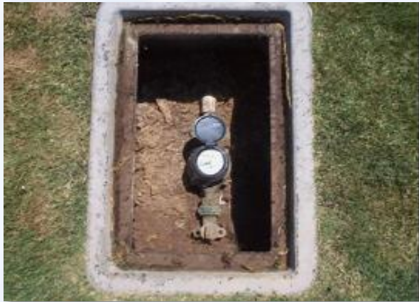
Install bulk water meters
