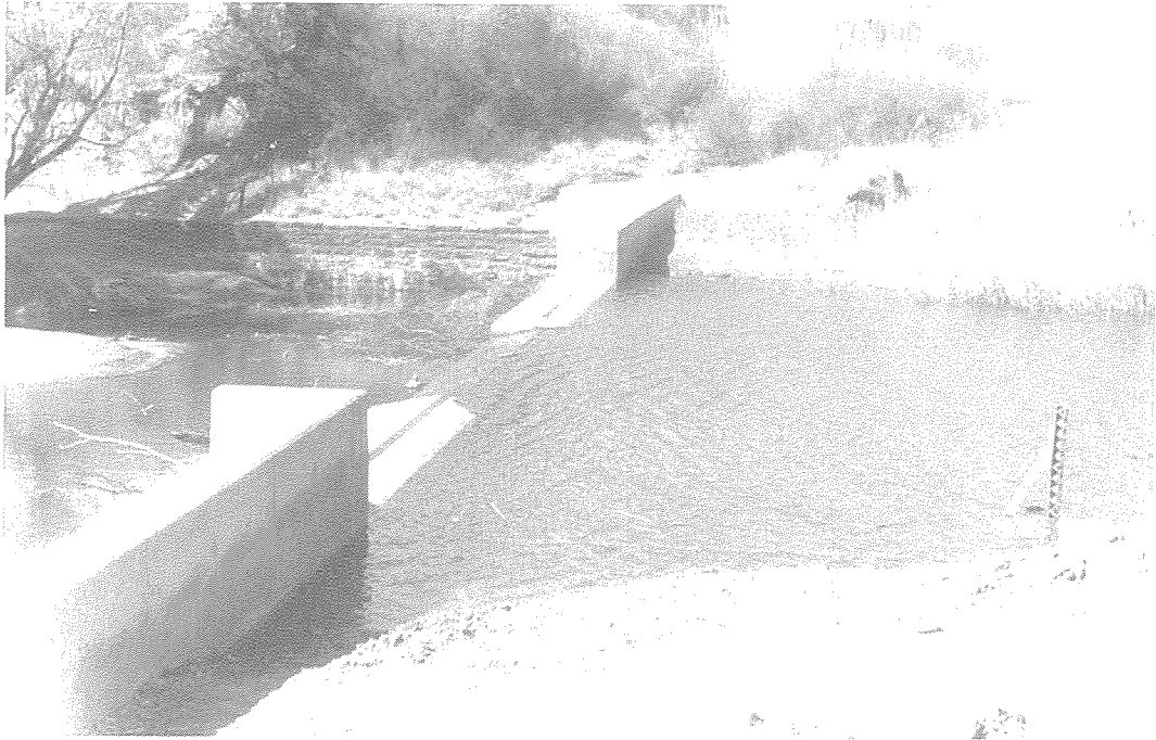
(a) Crump Weir Without Dividing Walls (C5 H003 Modder Rivier: Sannaspos)
