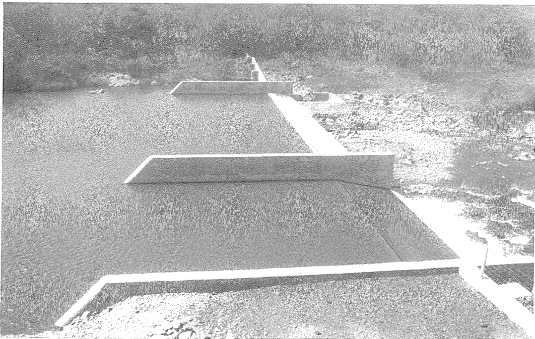
(b) Crump Weir With Dividing Walls (X1H001 Komati River: Hooggenoeg)
