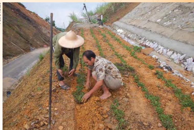
Community members construct bioengineering interventions to protect a roadside slope from erosion in Thai Nguyen, Vietnam.
