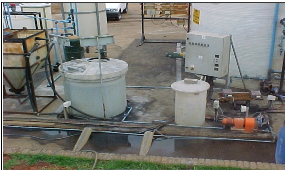
Photogram 4: Chemical Storage Tanks and Dosing Pumps
