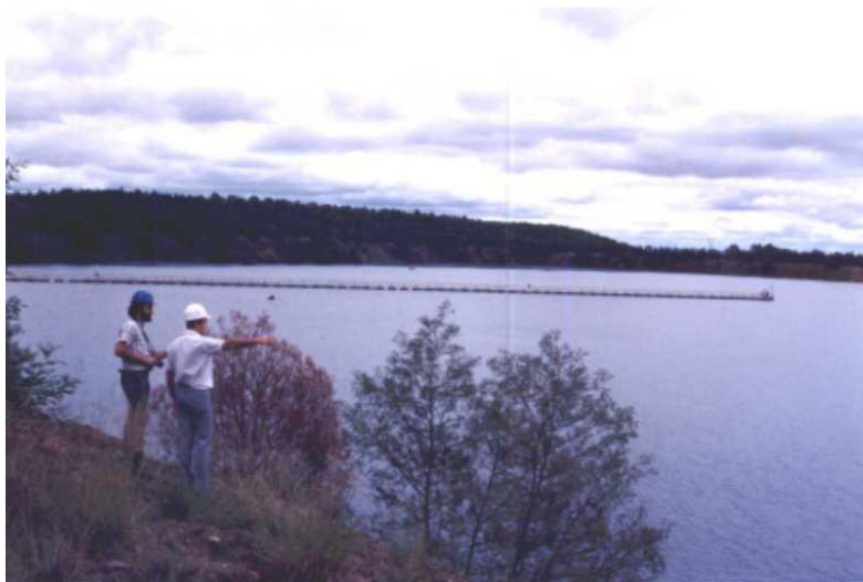
Figure 6 - Slimes Dam at Middelburg Mine Services
