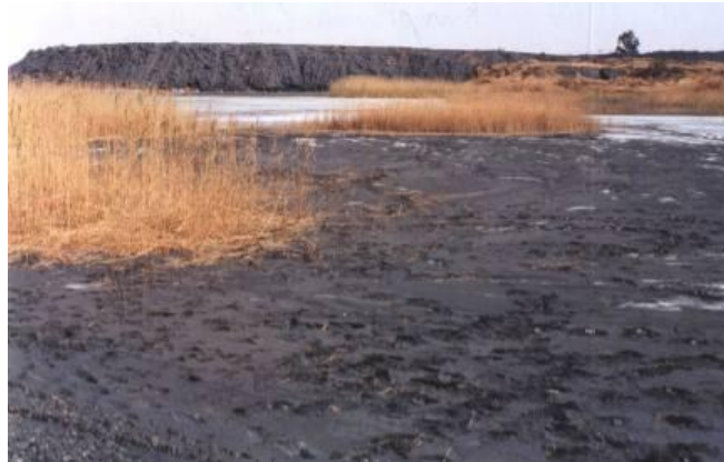
Figure 7 - Poorly Controlled Surface Slimes Dam
