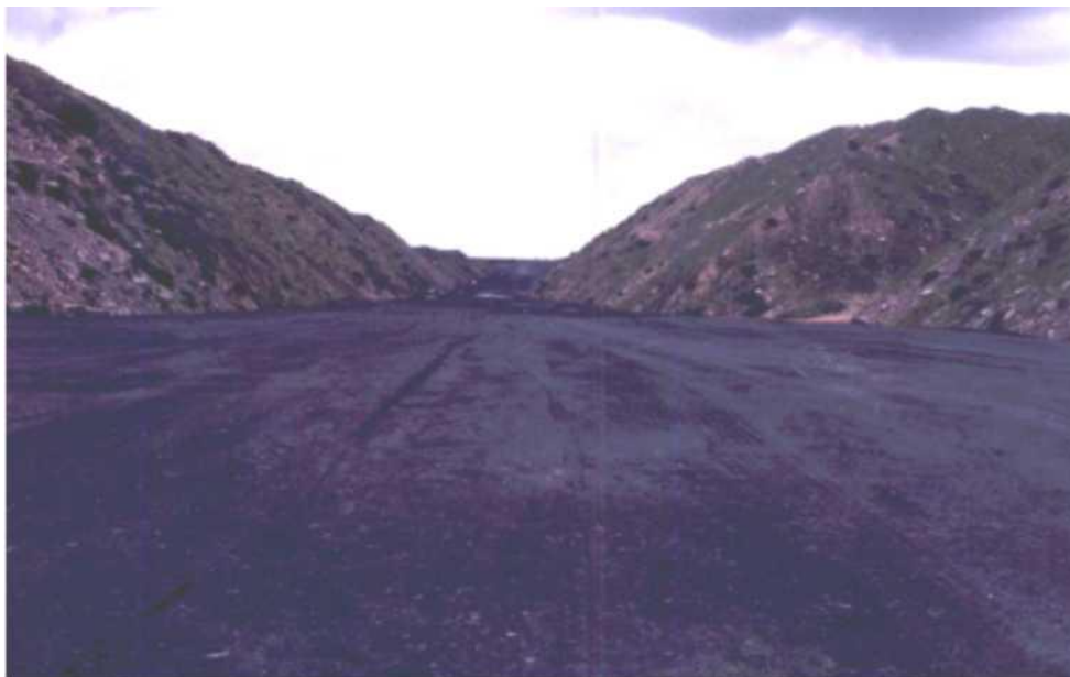
Figure 8 - Filling In Pit Voids
