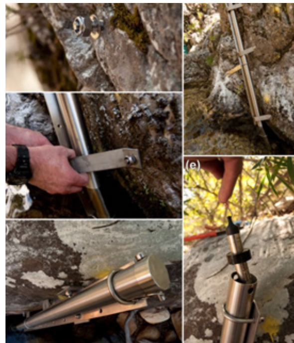
Figure 2. (a) Raw/bolt insertion into bedrock, (b) Fitting the mounting bracket to the mounting plate, (c) cap on the stilling well held in place with a bolt and clinch pin (d) installed stilling well with mounting brackets, (e) inserting the Solinst water level logger
