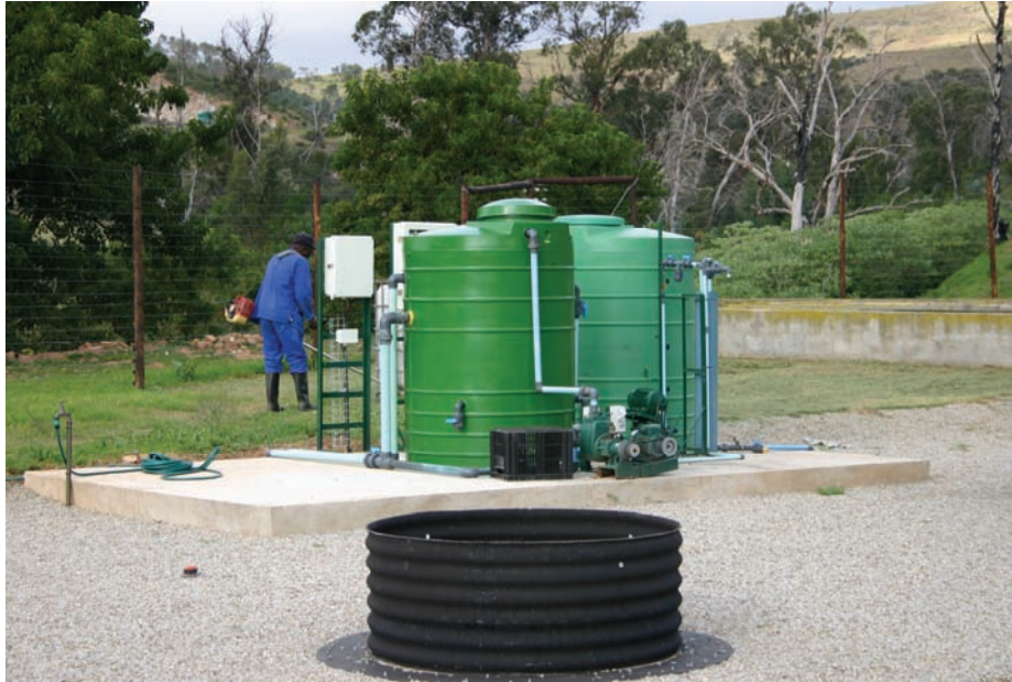
Figure 8: Blending tanks used for the make-up of the saline sewage fed to the saline IAPS system with the anaerobic pit of the Primary Facultative Pond shown in the foreground before its erection
