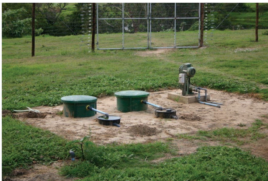
Figure 10: Algal biomass settling tanks and recirculation pump serving the High Rate Algal Ponds of the saline IAPS pilot plant
