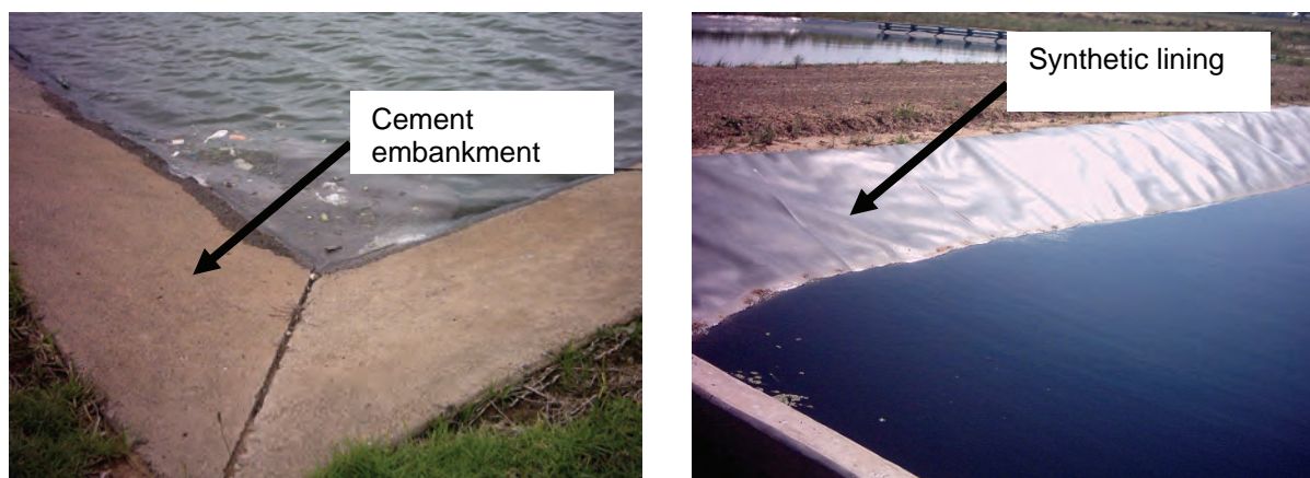
Figure 12: Photographs showing lining in ponds
