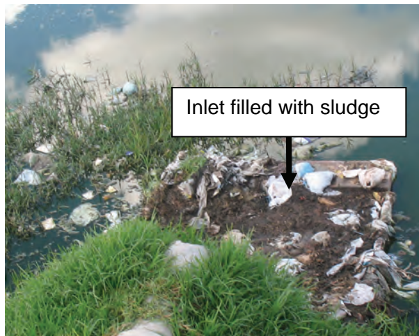
Figure 23: Sludge removal issues
