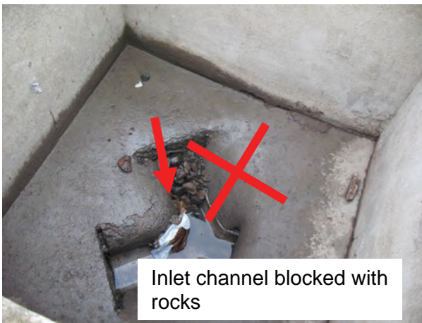
Figure 13: Inlet flow splitting device
