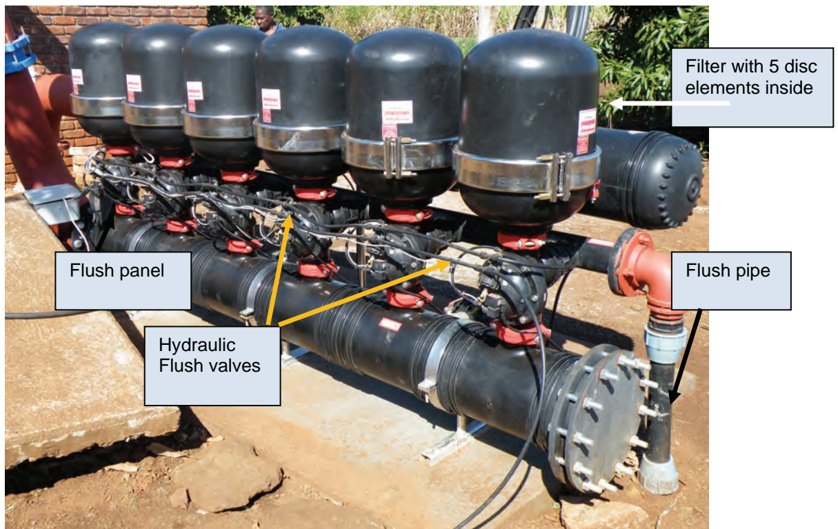
Figure 27. Arkal Spin-Klin® filter bank
