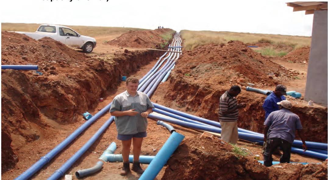
Figure 32. Laying of main lines from pump house
