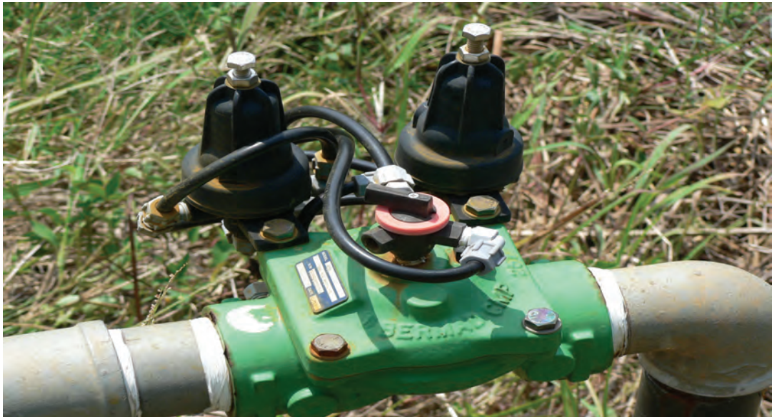
Figure 39. Pressure sustaining and control valve setting
