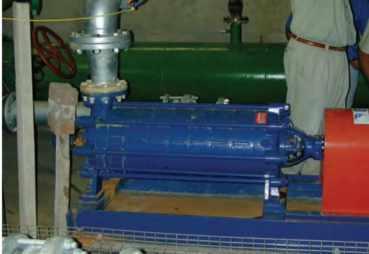
Figure 9. Multi stage pump (Multiple impellers)
