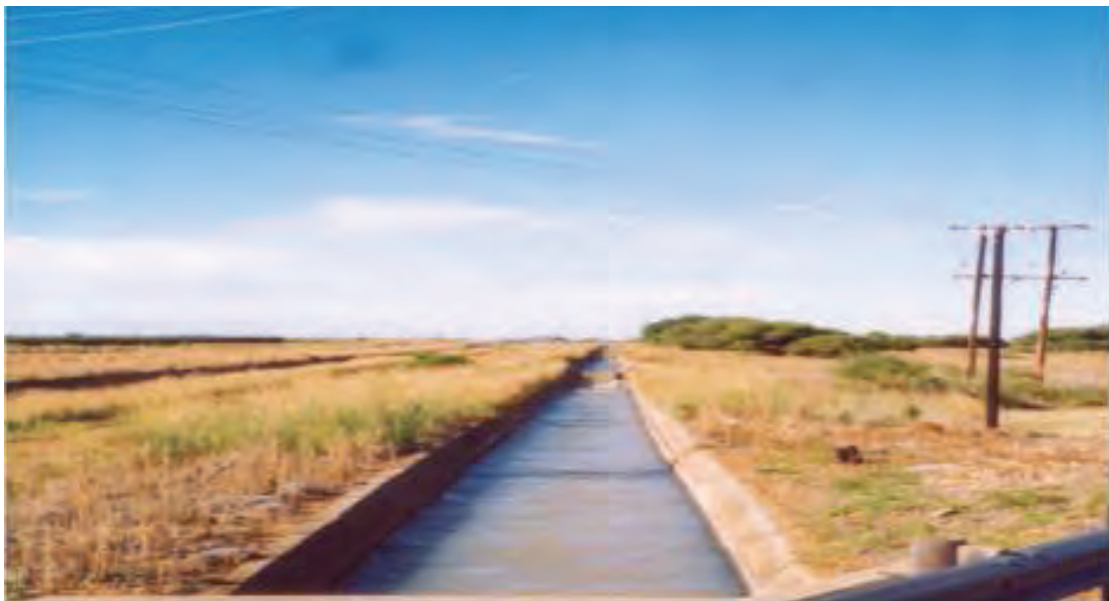
Figure 3. Canal water delivery system, Rietriver Irrigation Scheme
