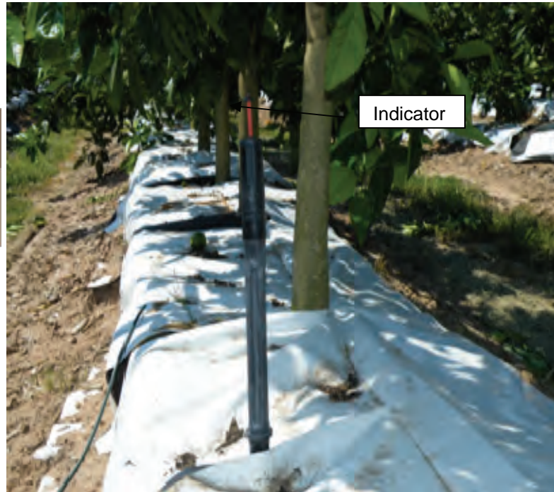
Figure 7. Installed wetting front detector in a citrus orchard
