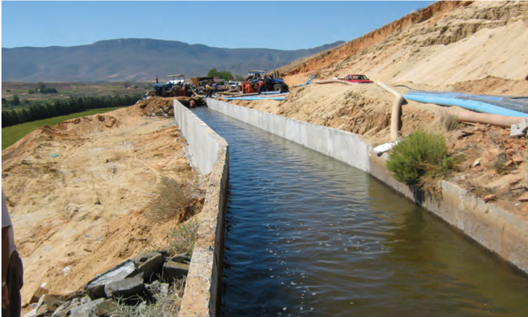
Figure 4. Canal water delivery system, Klaver Irrigation Scheme
