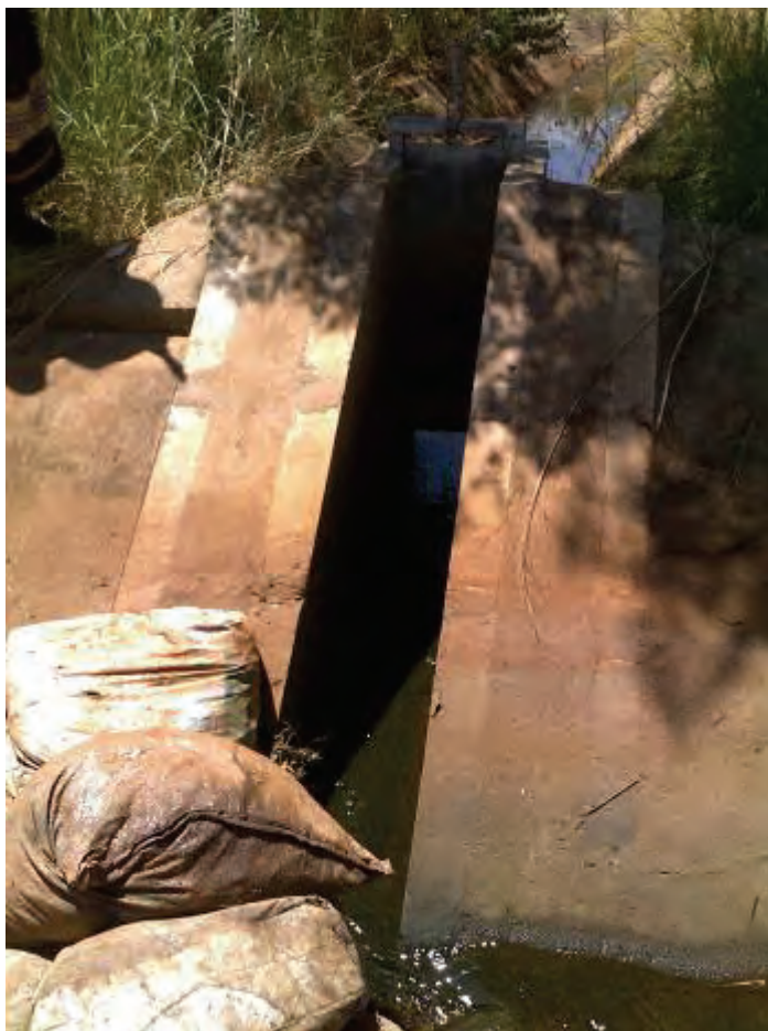
Figure 30: Sluice gate for the Hereford scheme small-scale farmers' water supply
