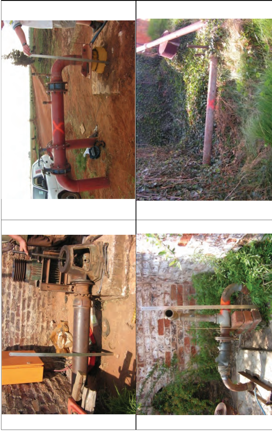
Figure 7: Typical boreholes to be fitted with meters
