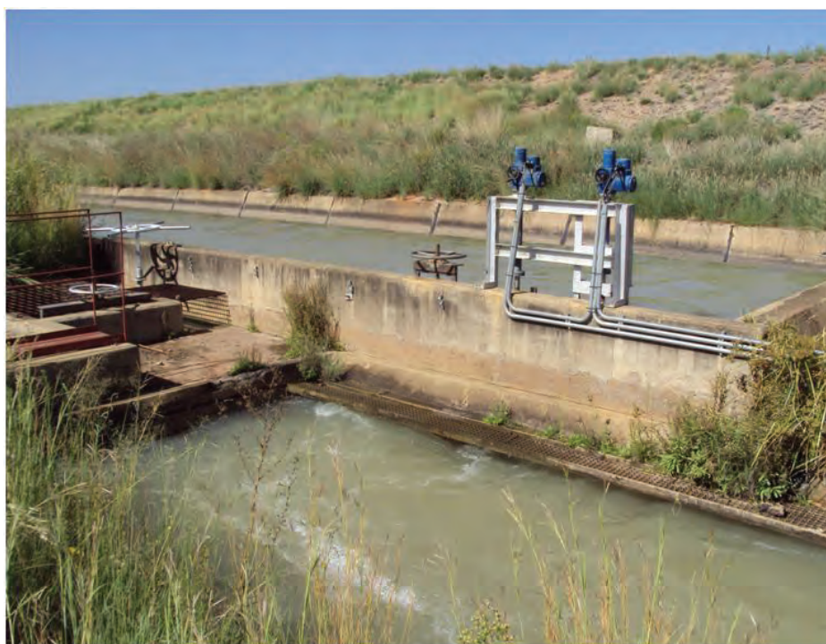
Figure 27: Automated sluice gates on the Orange-Riet scheme
