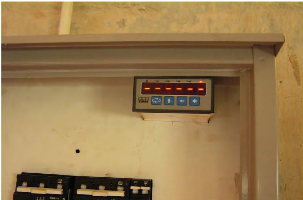
Figure 42: Display unit of the flow meters at Thabina Smallholder Irrigation Scheme
