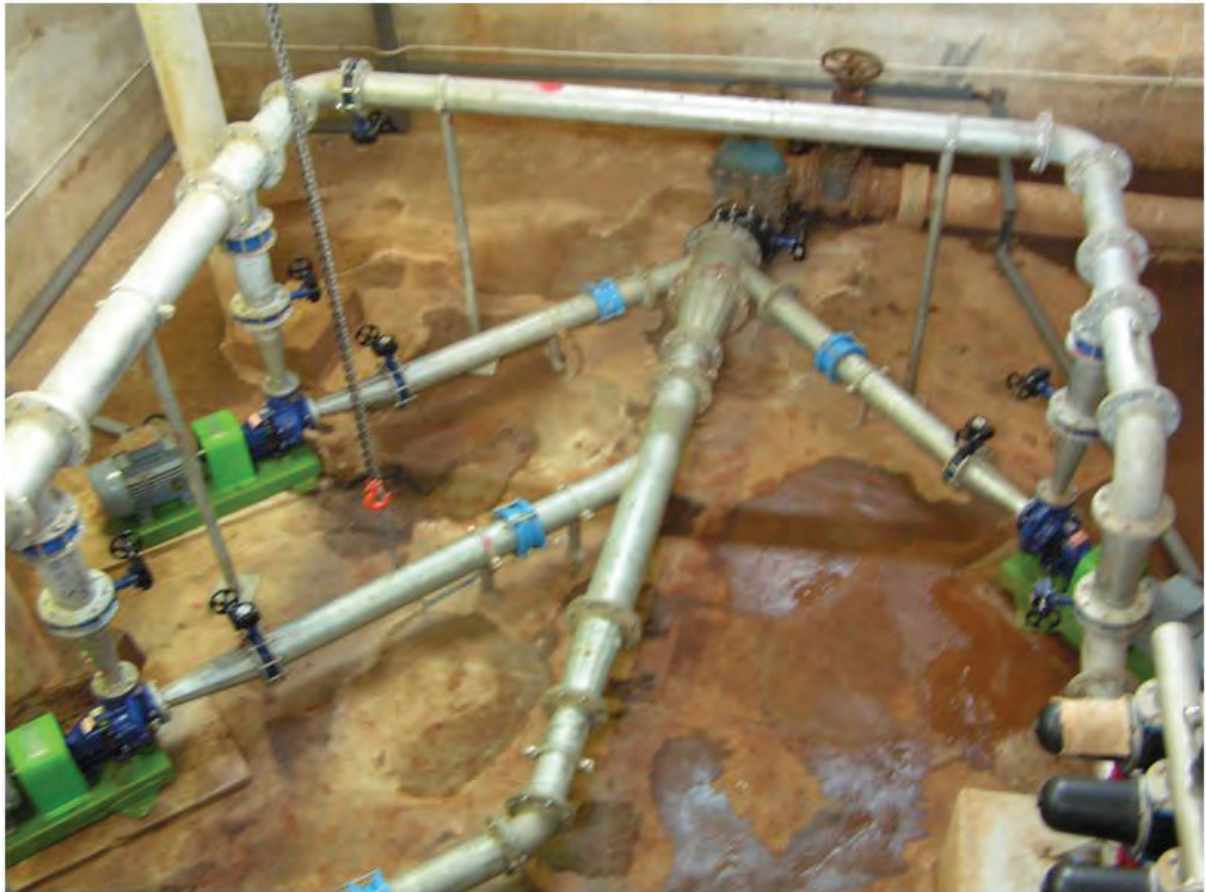
Figure 40: The new pump station at the Thabina Smallholder Irrigation Scheme
