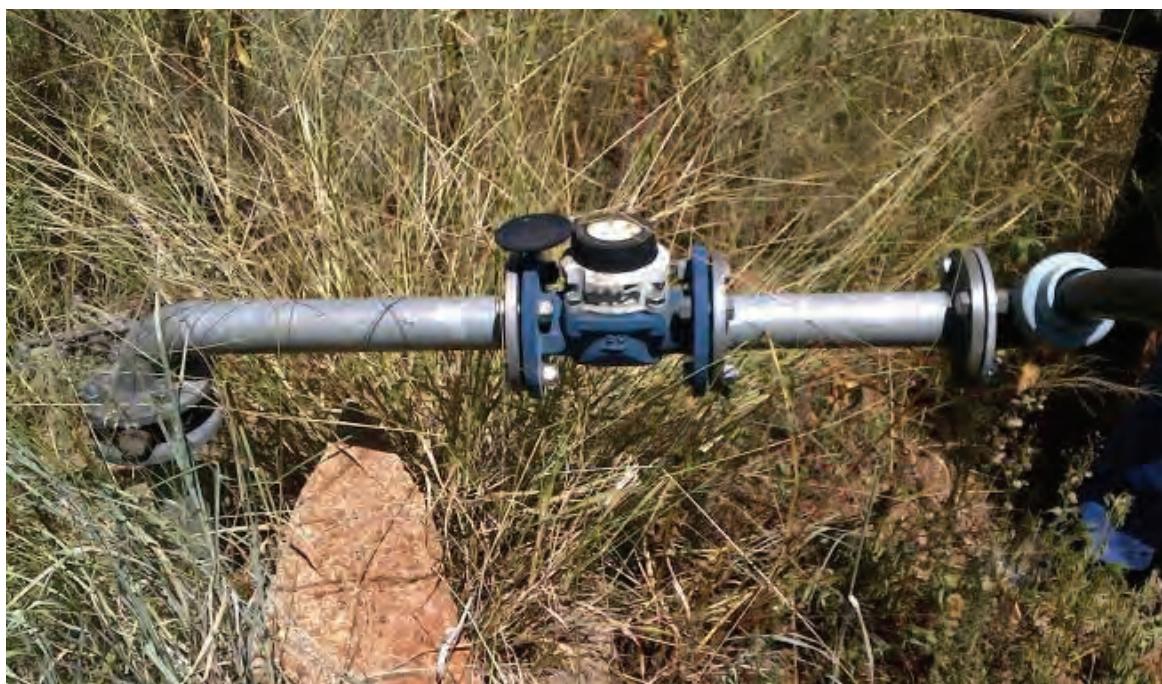
Figure 36: Farm hydrant with valve and water meter
