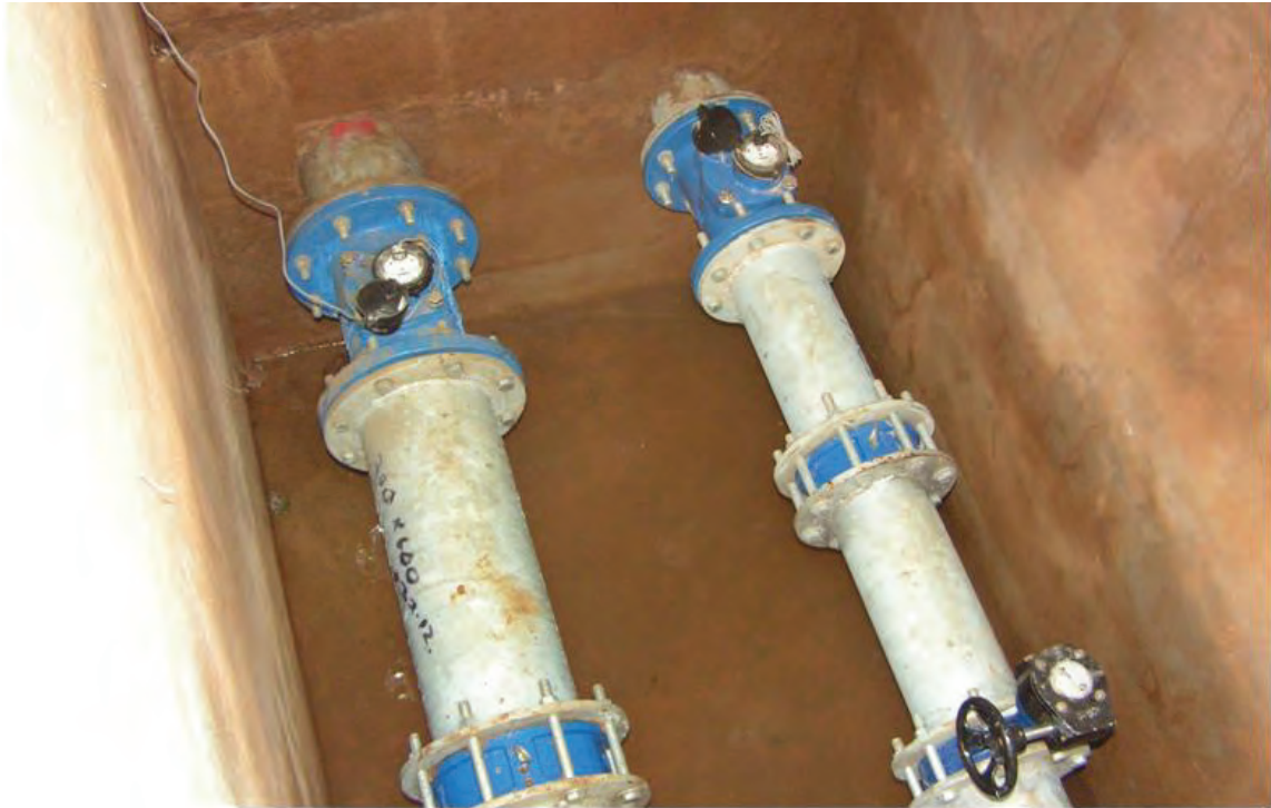
Figure 41: Flow meters installed at the Thabina Smallholder Irrigation Scheme
