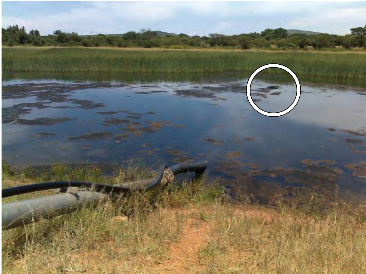
Figure 34: Float-mounted pump suction pipe withdrawing water from dam
