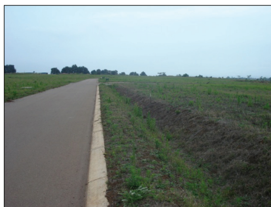
Figure 4.2: Roadside swale, Cotswold Downs Golf Estate, Hillcrest
