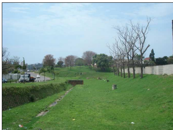
Figure 5.1: Large roadside detention pond, Hillcrest
