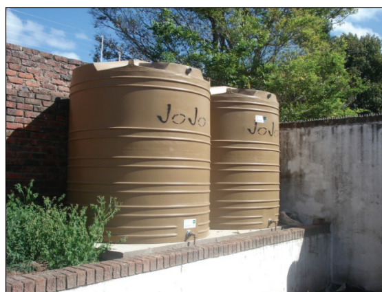
Figure 3.4: Roof runoff storage tanks for household purposes
