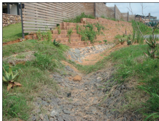
Figure 4.4: Gabion-lined dry swale, Hawaan Estate, Umhlanga
