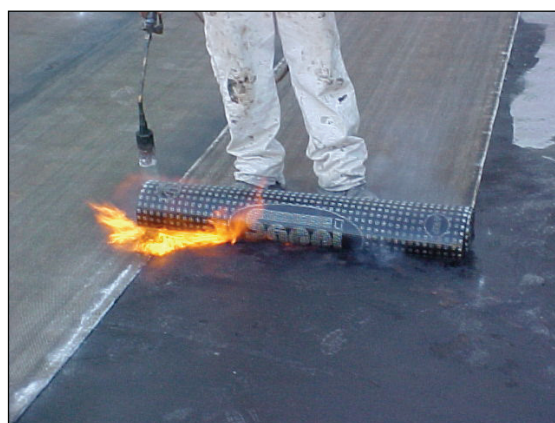
Figure 3.2: Waterproofing a roof in preparation for the construction of a green roof
