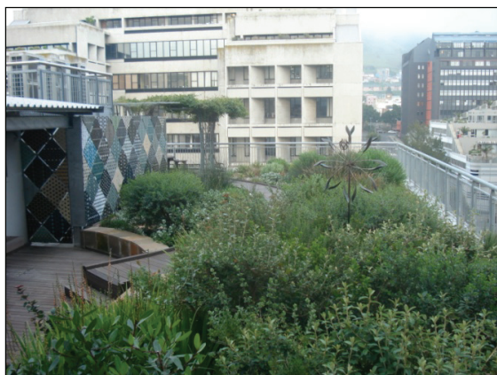
Figure 3.3: Intensive green roof, Department of Environmental Affairs and Development Planning, Cape Town
