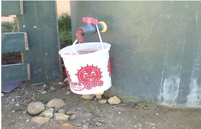
Figure 2-5: Measures implemented to prevent water wastage, where DRWH tank taps were leaking.
