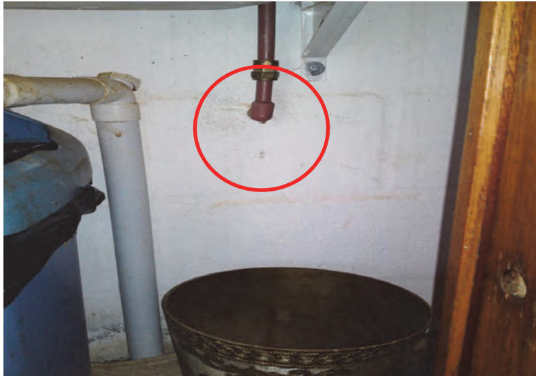
Figure 2-13: Photograph of a leaking pipe inside a kitchen with a bucket to collect the water drops.
