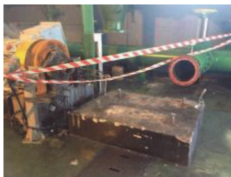
Plate B) Missing pump
