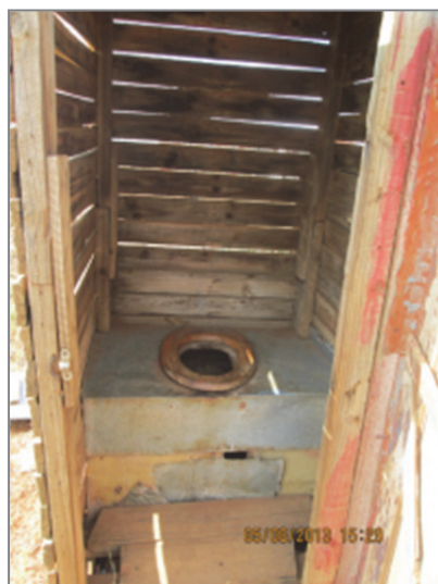
Figure 43 A self-made pit latrine, Orange Farm
