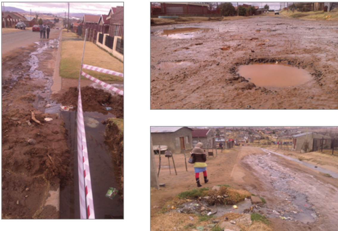
Figure 50 Flooded roads due to burst pipes or leaking infrastructure, Ficksburg
