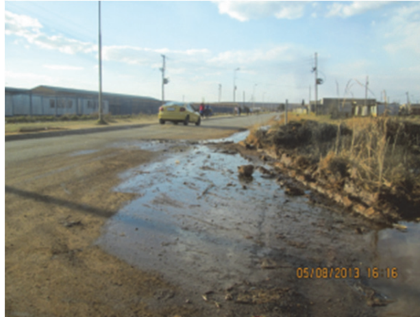
Figure 41 Flooded road due to burst water pipe, Orange Farm
