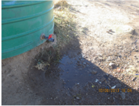
Figure 46 Jo-jo tanks' taps not positioned at the very bottom of the tank contribute to contamination of water
