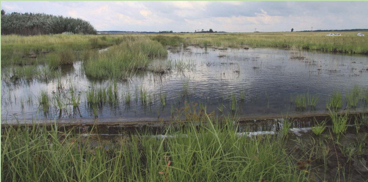
A view upstream of one of the rehabilitation structures in the Zaalklapspruit wetland. Reduced flow rates and diffuse, rather than concentrated flows have contributed significantly to addressing water quality impacts caused by AMD.
