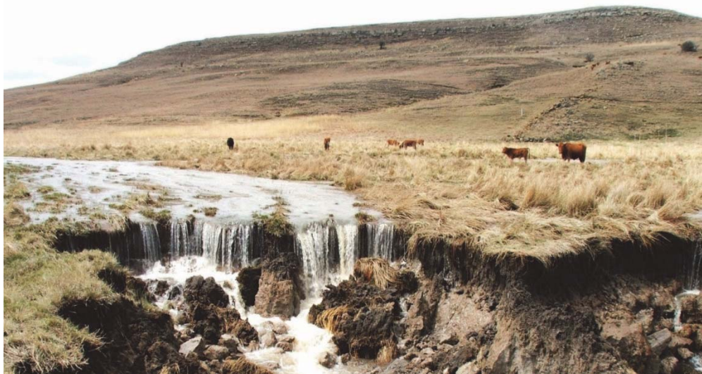
Wetland in a grazing landscape that is being severely eroded through head-cut advancement.
