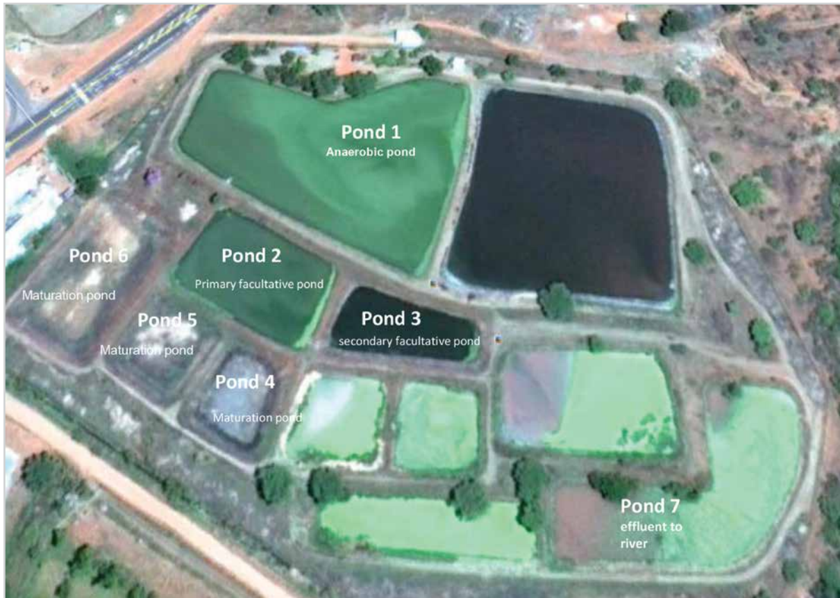
Figure 1: The Motetema Wastewater Treatment Works consist of four types of stabilisation ponds, namely (1) anaerobic pond, (2) primary facultative pond, (3) secondary facultative pond and (4) aerobic (maturation) ponds
