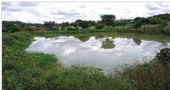
Figure 5: Water depth too low, causing rooted plants to invade pond
