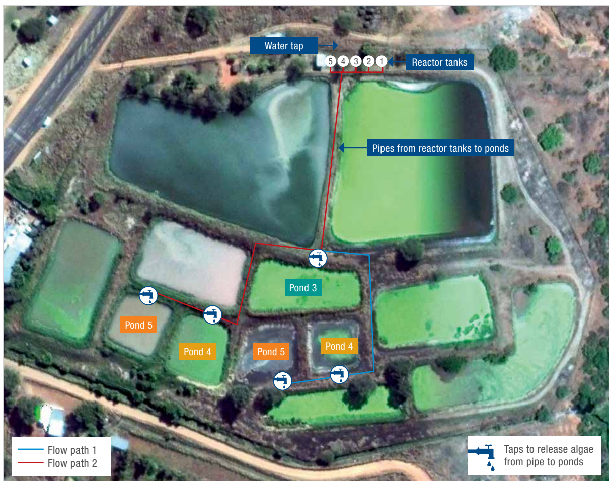
Figure 2: Lay-out of the ponds at the Motetema Wastewater Treatment Works, indicating the piping from the reactor tanks and the ponds to be dosed
