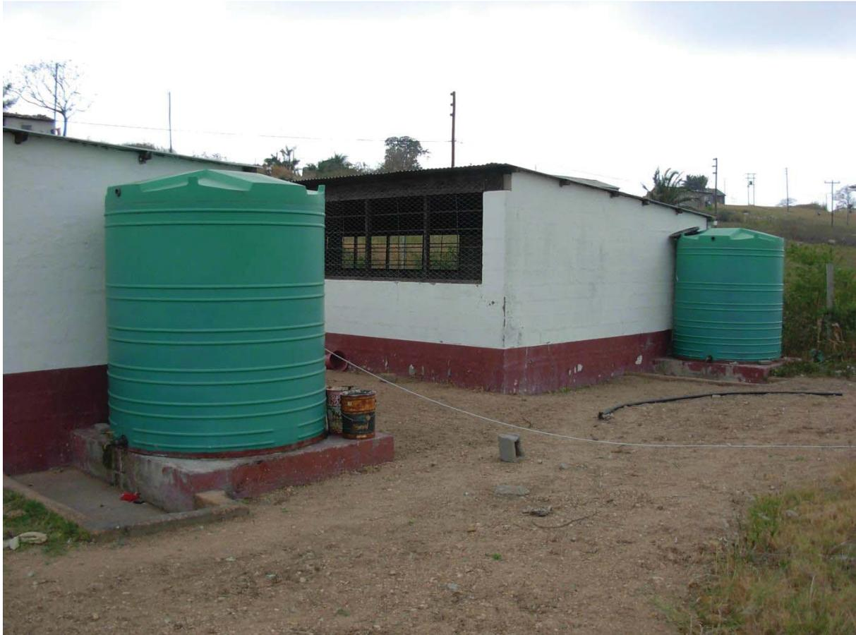
**Figure 2.1: Micro-catchment rainwater harvesting and storage from rooftop rainwater**
