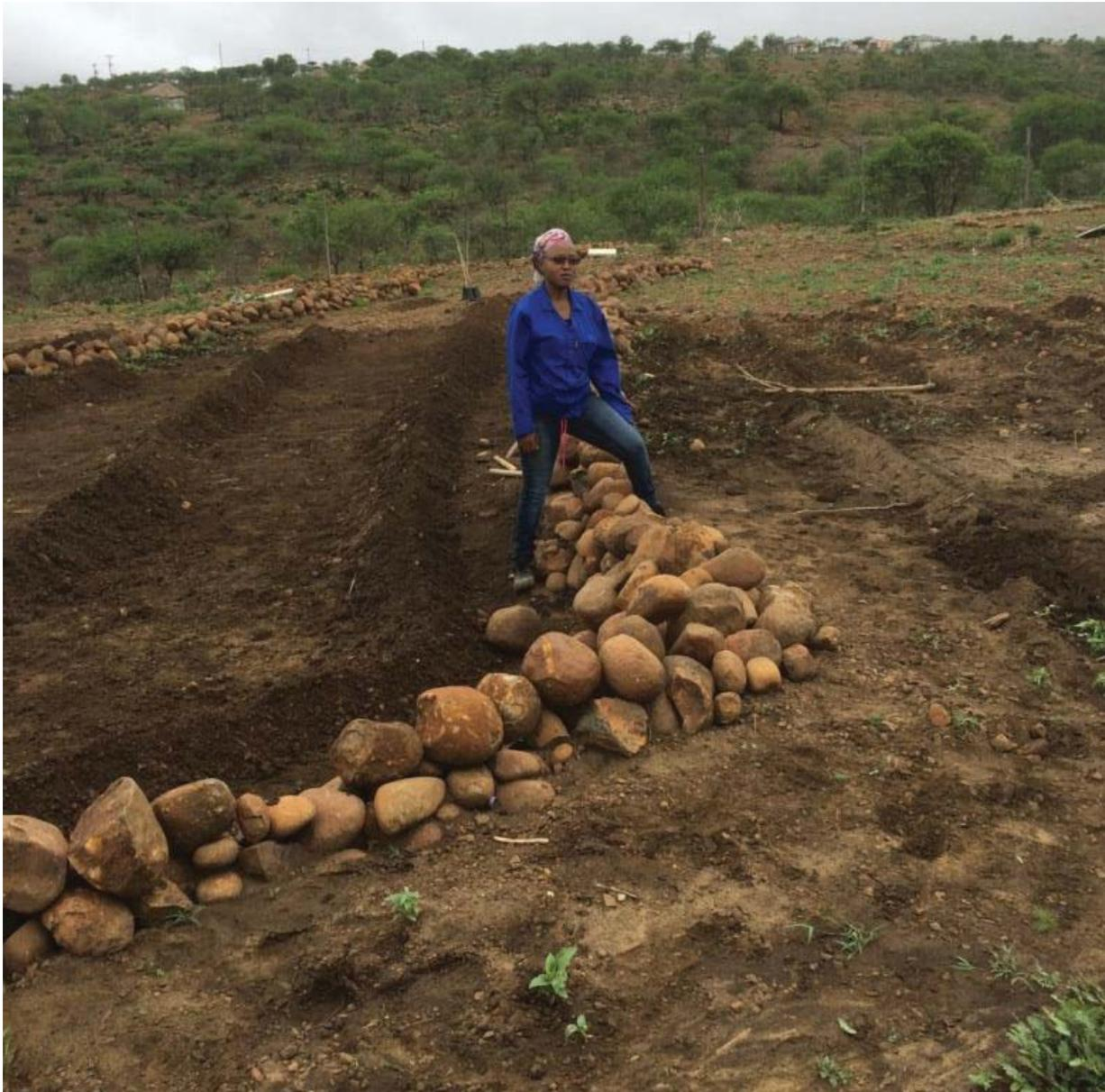
**Figure 5.26: Sediment deposition behind stone contour bunds at Mxheleni, Muden**
