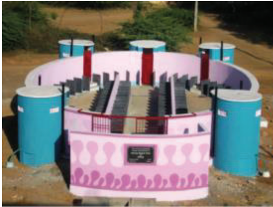
Figure 21: The completed sanitation facility at Valadore Girls' School, providing approximately 90 spaces for urination and 5 ecological toilets for defecation
