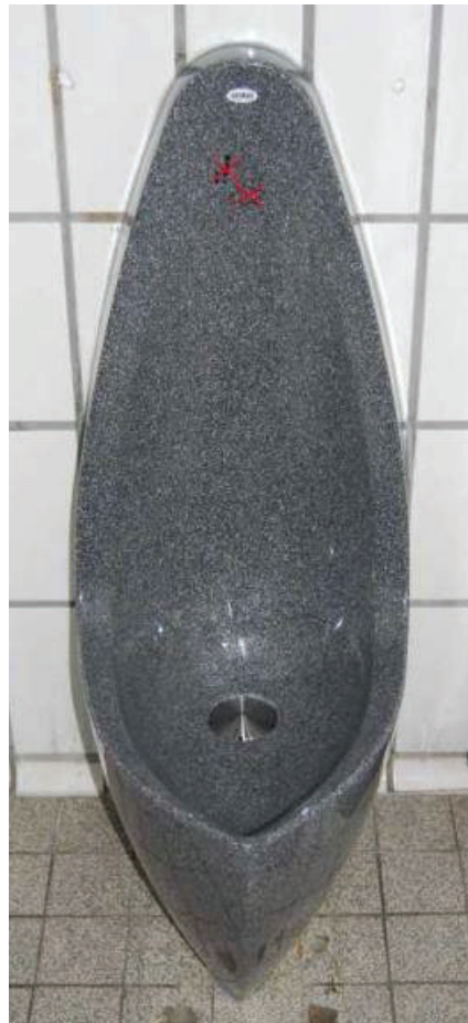
Figure 7: Example of a female wall mounted urinal with space to straddle and squat or stand ("Female Urinal Tested in Europe," 2012)
