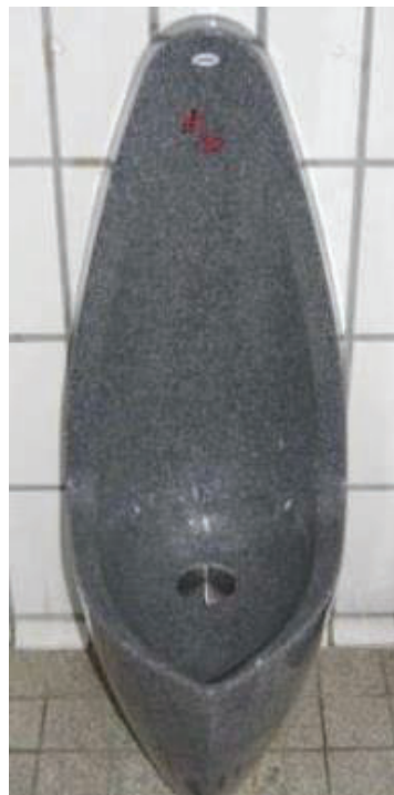
Figure 15: Female urinal developed by Uridan and used in Germany and India (“Female Urinal Tested in Europe,” 2012)
