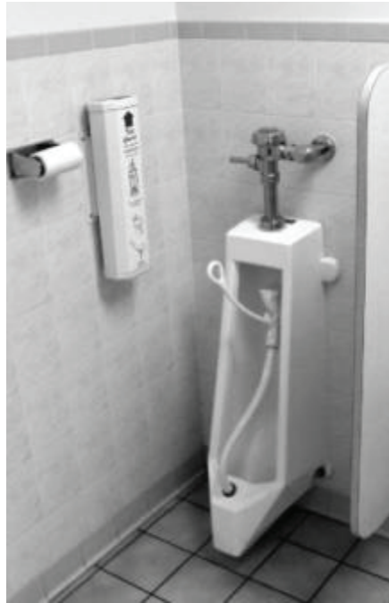
Figure 11: A She-inal installed in a Dairy Queen restaurant in Port Charlotte, Florida (Pohlen, 2003)
