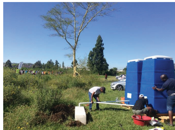
Figure 38: In some cases, a small hole had to be dug to ensure that the tank was below the outlet of the units
