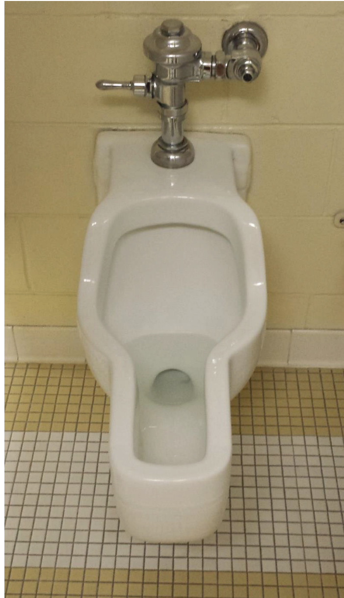
Figure 8: Photograph of a Sanistand from between 1964 and 1967 installed in a university dorm ( http://rebrn.com/re/iff-im-staying-in-a-dormitory-in-the-us-built-in-the-s-and-there-626706/ )
