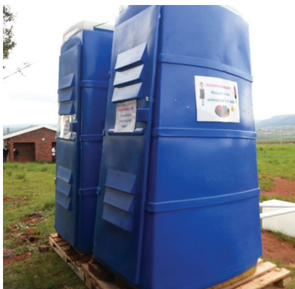
Figure 33: Two rectangular huts for the Weestands, sitting on pallets to provide necessary height for drainage of urine
