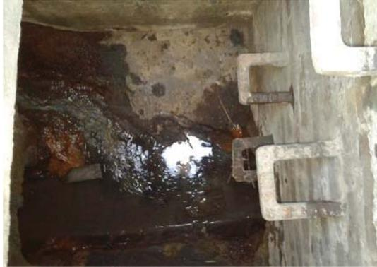
**Figure 5-11: Photo of illegal discharge in manhole 17CHA**
