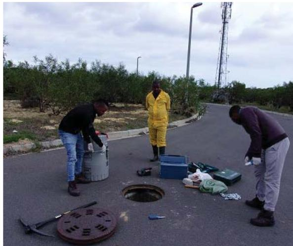
**Figure 4-6: Isco 6712 Portable Sampler – installation in a manhole**
