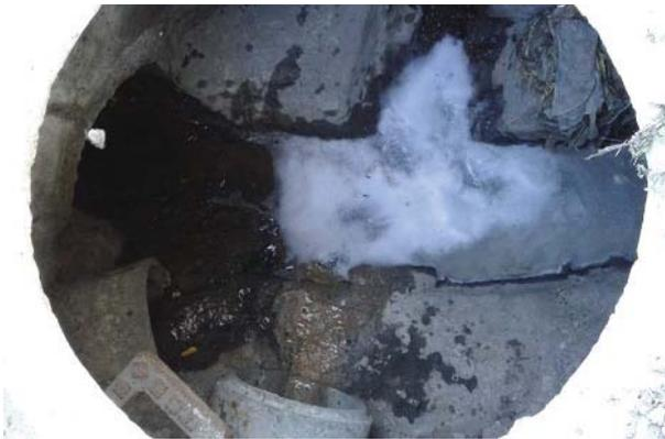
(c) Manhole 7ALT with white soapy foam discharge. (d) Stormwater inlet with stain.
