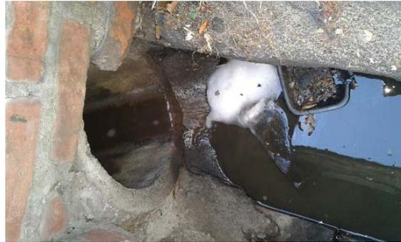
**Figure 5-7: Car wash effluent discharging into manhole 19MON**
