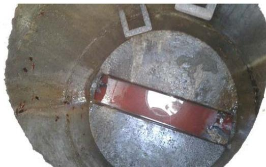
**Figure 5-10: Photo of deep maroon colour discharge in manhole 4FOU**
