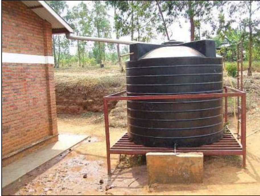
Figure 2-6: Rooftop rainwater harvesting technique for the collection of rainwater from roof surfaces, with subsequent storage in tanks connected to gutters adjacent to roofs. Water stored in tanks is used for irrigation of small gardens (Source: Castelo, 2018).
