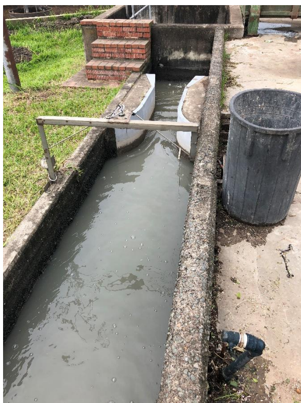
Figure 9: Evidence of no flowmeter at KwaDukuza WWTW (i.e. no flow measurement)
