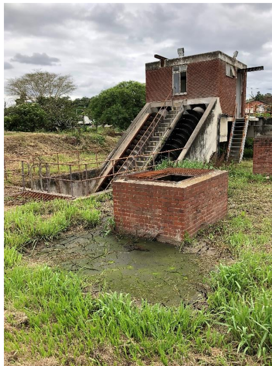
Figure 10: Evidence of previously overflowing units at KwaDukuza WWTW
