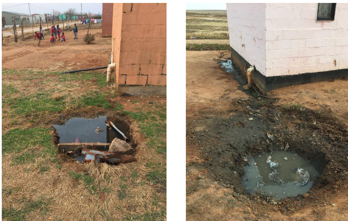
Figure 7: Evidence of full and overflowing containment tanks
