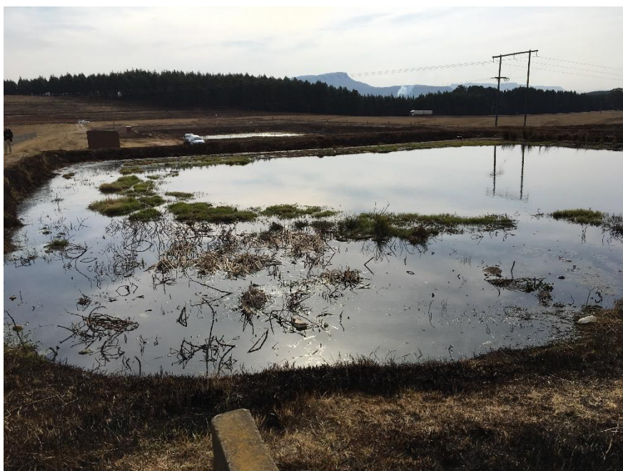
Figure 12: Ugie Ponds showing accumulated sludge
