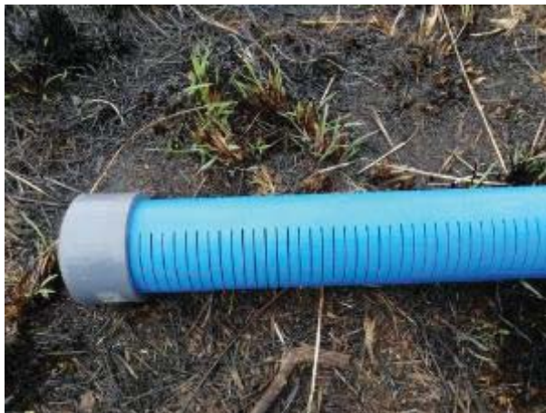
Figure 2: Left: The capped end of the 1 m length (50 mm diameter) slotted pipe that provides for the below-ground offtake of water from the spring. Right: The fittings linking this slotted pipe to the main pipe (50 mm HDPE) (from Chris Stimie – RIEng).
