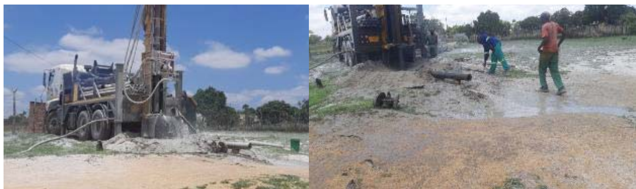
Figure 13: Left: The drilling machine. Right: Water starting to flow during the drilling process.
