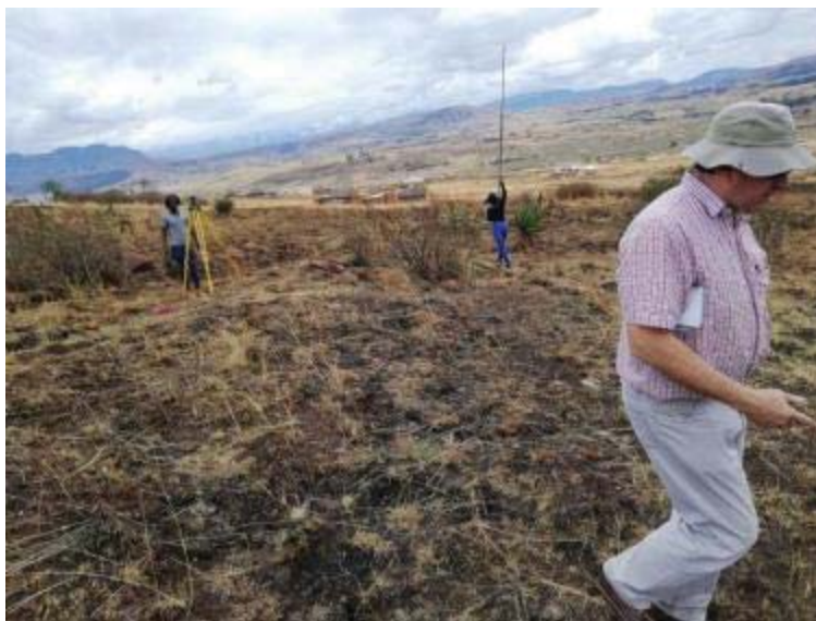
Figure 4: Left: measuring the gradient for the main pipeline using a dumpy level. Right: Adjusting the line for the pipe to avoid some of the larger dongas and rough terrain, while keeping it on an even gradient.
