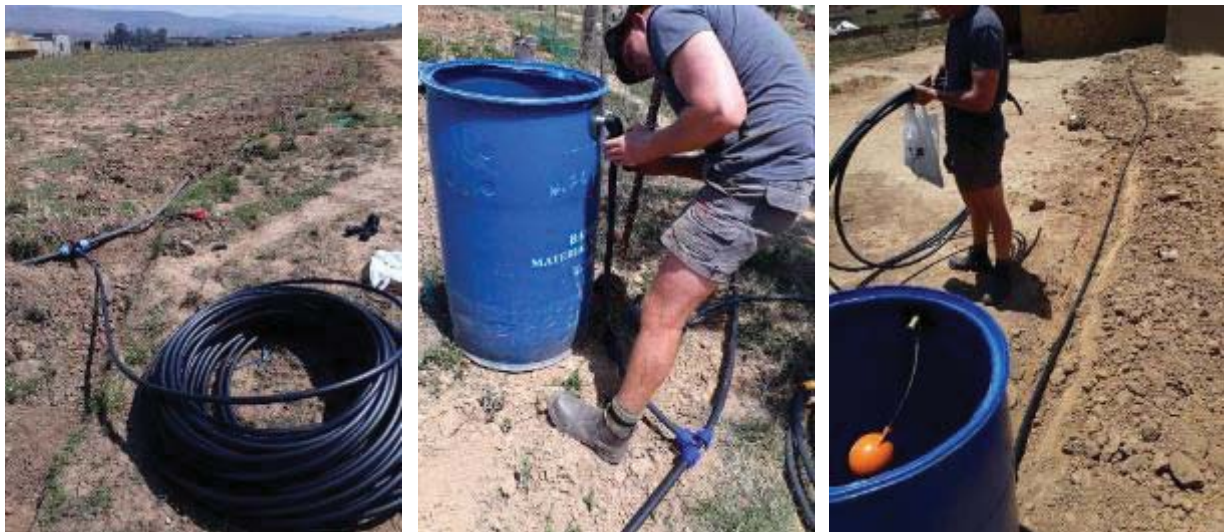
Figure 8: Left to right: Laying the piping along the edges of the fields. Pipe branches towards the different homesteads. Fitting the inlet pipes to the 200 L drums. Installation of a float valve in each drum.
