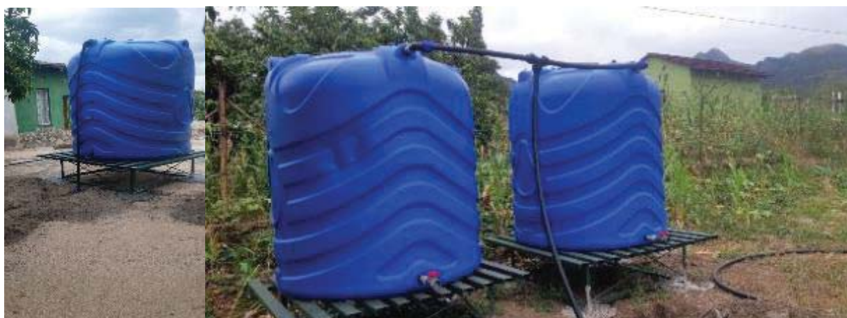
Figure 23: Left: Header tank at Sedawa (Joyce Seotlo). Right: Header tanks (4 500 L each) fully functional and tested at Turkey (Michael Makgobatlou).
