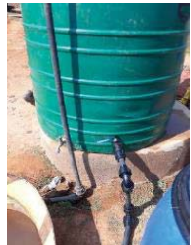
Figure 7: Plinth for the 2 200 L header tank
