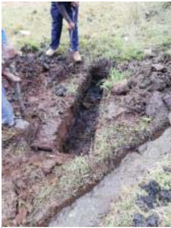
Starting on the trench for the slotted pipe, below the spring and pond
