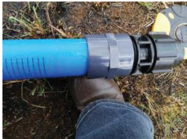
Figure 2: Left: The capped end of the 1 m length (50 mm diameter) slotted pipe that provides for the below-ground offtake of water from the spring. Right: The fittings linking this slotted pipe to the main pipe (50 mm HDPE) (from Chris Stimie – RIEng).
