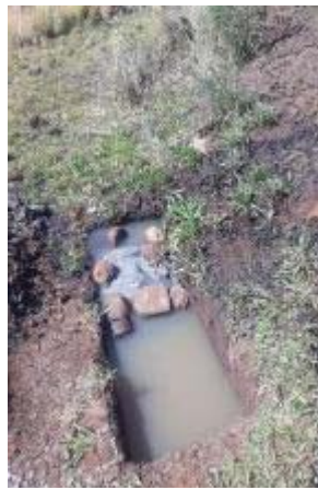
The trench with slotted pipe installed in a bed of gravel, covered by shade cloth and rocks with a small furrow leading water from the spring to this trench
