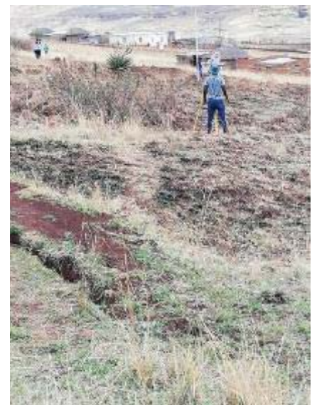
Figure 4: Left: measuring the gradient for the main pipeline using a dumpy level. Right: Adjusting the line for the pipe to avoid some of the larger dongas and rough terrain, while keeping it on an even gradient.
