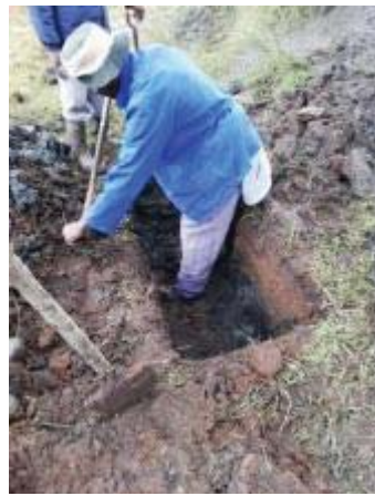
Deepening and widening this trench to 50 cm x 50 cm x 1,2 m
