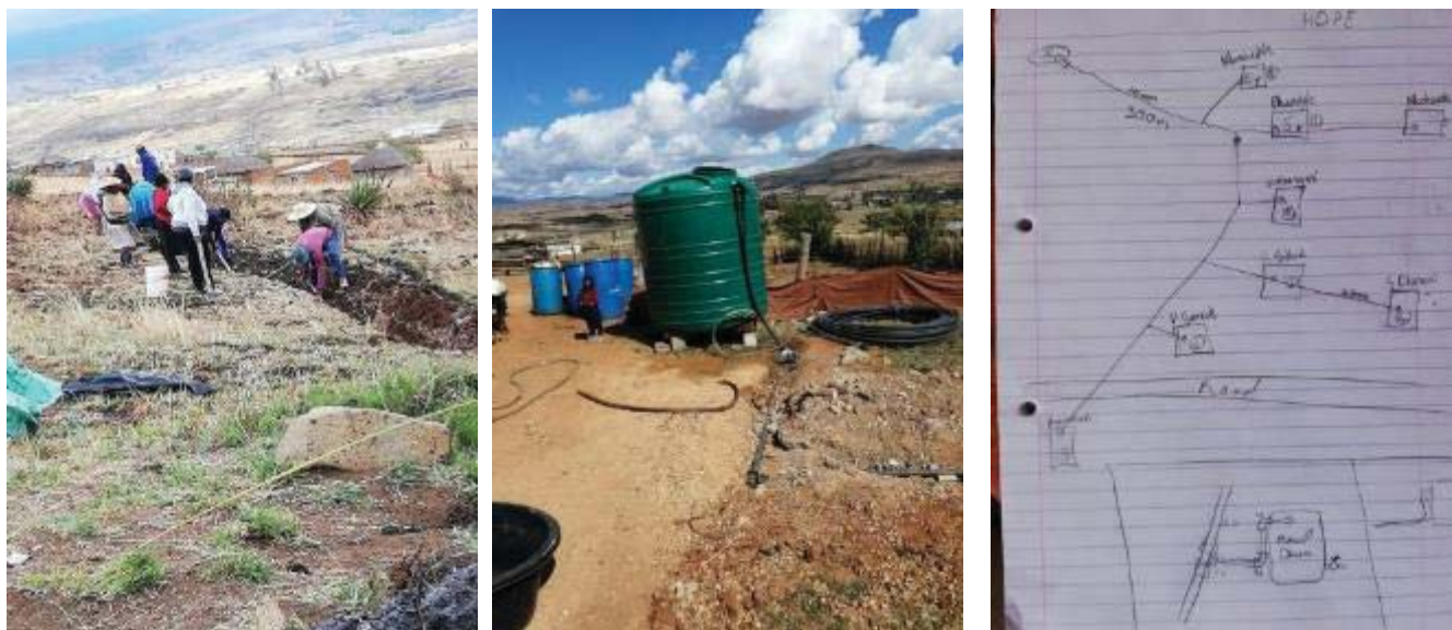
Figure 5: Left to right: Group members digging the ditch from the spring to the header tank. The header tank at Phumelele Hlongwane's homestead – which was not installed on a level platform and has subsequently been corrected. Initial rough layout drawing of the flow of the water to participants' homesteads.
