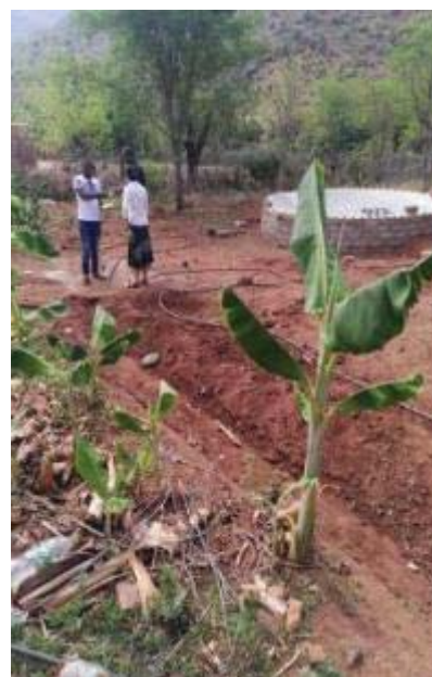
A completed geofabric tank with brick wall and roof for safety. The inlet furrow for water is in the foreground
