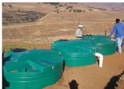
Partially buried Jo-Jo tanks for harvesting water off slopes
