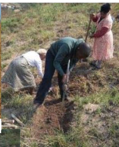
Digging the ditch for keying in the stones for the check dam
