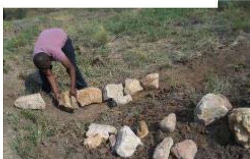
Starting to pack the check dam. Large rocks go at the bottom
