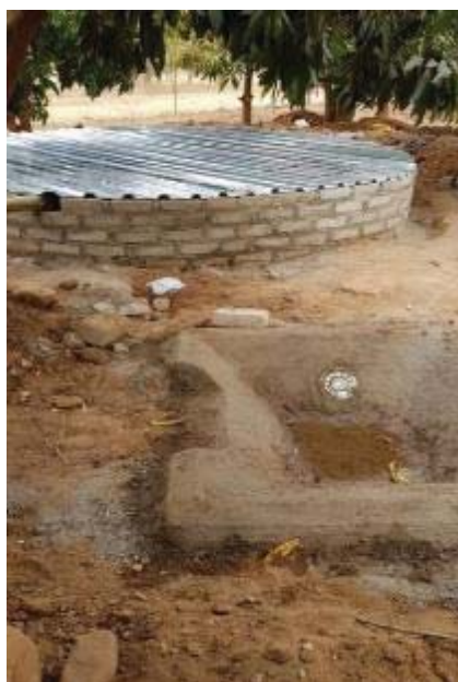
The silt trap for a 25 000 L underground tank to reduce silt load of stored water
