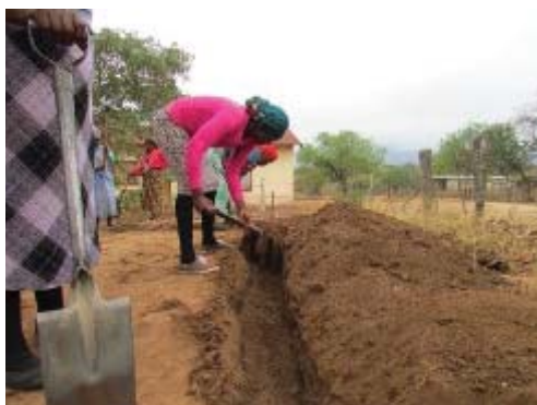
Digging a diversion ditch (1,5-5% slope; 30 cm wide and 30 cm deep with soil placed on upper slope
