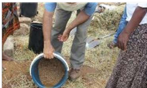
Both the gravel and sand is rinsed prior to use, to make sure they are clean and to avoid clogging up of the system (2015)
