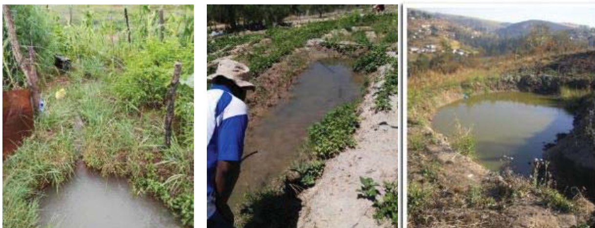
Three examples of small dams/ponds dug in soil that will hold water — >25% clay to be sure. The one on the right is a 'large' dam fed by a spring slightly higher up the slope. The dam in the central picture is fed by a pipe gravity fed from a river
