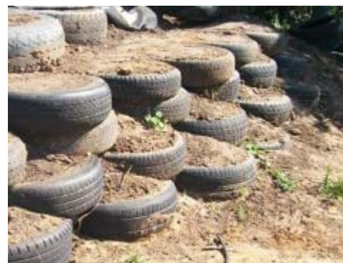
Terraces can also be built using old tyres in areas where stones are scarce
