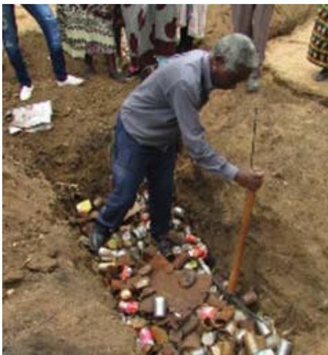
Trenches are dug 60 cm-1 m deep. The bottom layer is made up of old tins or branches
