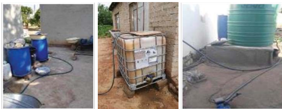
Local RWH storage options in Limpopo; basins, 210 L drums, 1000 L containers and Jo-Jo tanks, these hold little water
