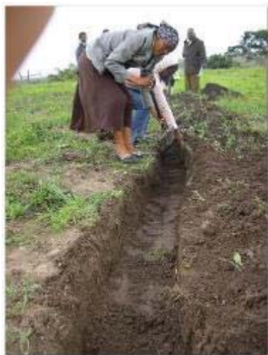
Digging the cut off drain/swale ditch. Soil is placed on the downslope
