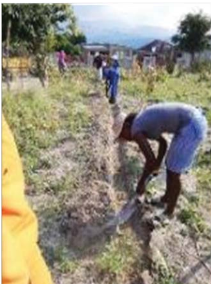
Digging out a shallow trench 30 cm wide and 15 cm deep on a contour line in a
