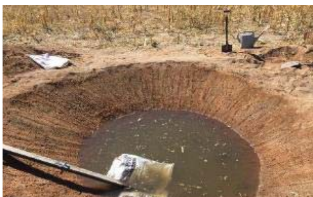
A small pond lined with bentonite (the yellowish clay inside the pond,) being filled up. Note the angle of the pond walls, the slope of the pond walls, that allows for the bentonite to be stamped into sides and bottom of the pond to seal it.
