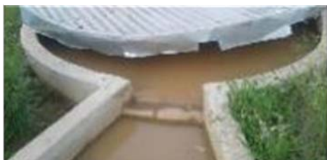
An example of an underground tank (18 m 3 ), with a removable metal roof (Acornhoek).
