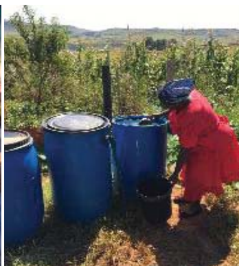
An example of a household connection. These drums are interlinked and have a float valve to ensure the water stops running when the drums are full
