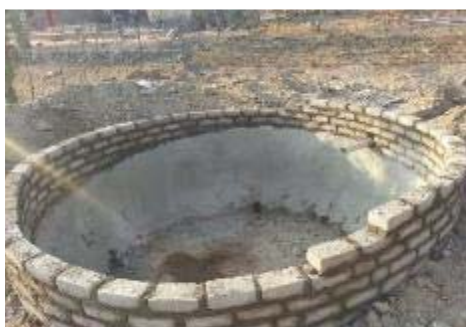
A ferrocement underground tank with brick wall for placement of a roof structure under construction
