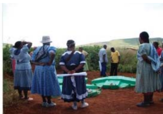
Jo-Jo tanks buried for underground water storage
