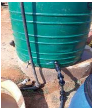
An example of a header tank from where water is gravity fed to the households
