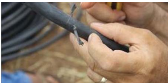
Holes are made through the dripper pipe, from side to side and some plastic string is threaded through the holes and tied with knots to create the "drippers"
