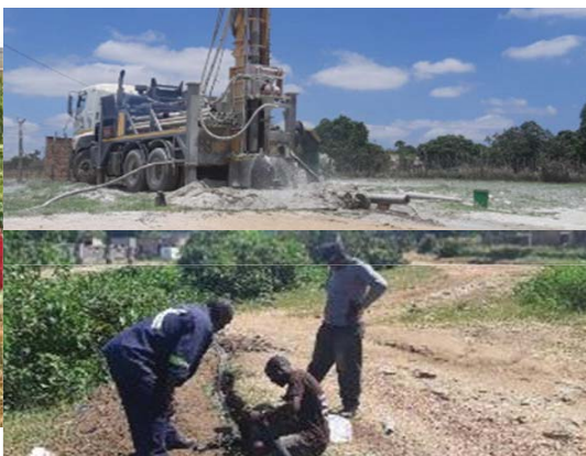
Drilling of boreholes and laying of pipes from the header tank to the households
