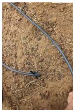
The pipe is sealed at the end by bending it over and clamping it
