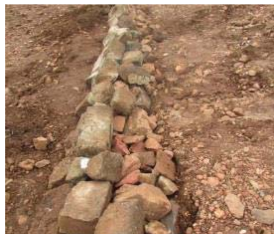
A view showing the stones keyed into a ditch with larger stones downslope of the smaller stones.
