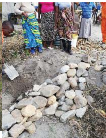
An example of a completed check dam with the apron below the wall and the banana shape of the wall visible.
