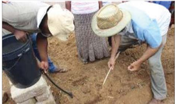
The bucket is placed on a stand and a down pipe is connected, to ensure there is pressure in the dripper lines
