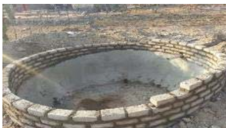
Ilthangi leferrocement eligujelwe ngaohansi elinodonga lwezitini ukwakhela indawo yokubamba amanzi nophandla osusakhiwa
