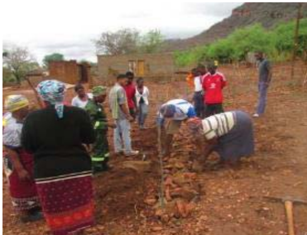
Stone lines- akhiwa phezu kwekhontolo kanti angenzinwa endaweni noma engakanani
