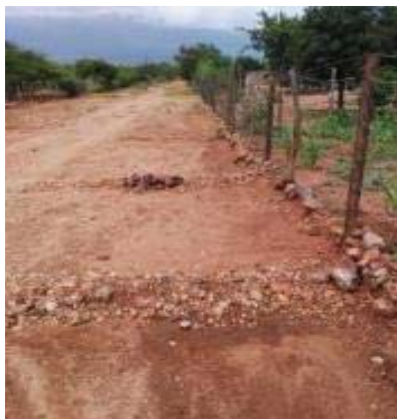
Amatshe amancane asebenzisela okulawula ukugeleza kwamanzi emgwaqeni awahambise ezingadini
