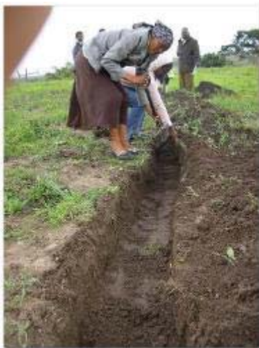
Ukumbiwa kwe -swale inhlabathi ibekwa ngasohlangothini olwehlelayo
