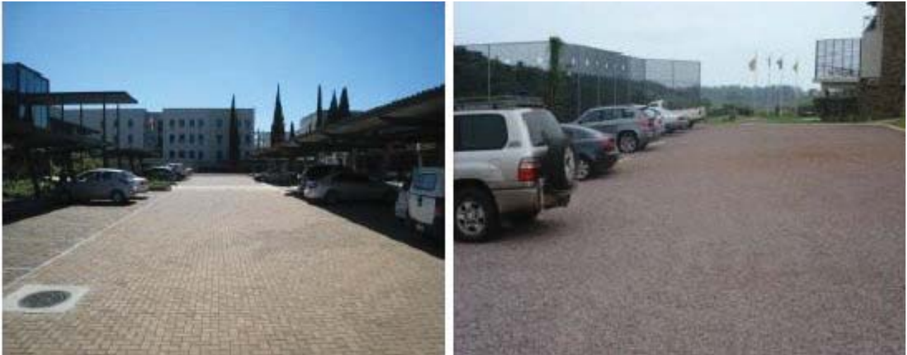
Figure 37: Pictures of Stellenbosch (left) and eThekweni (right). These are some examples of where semi-permeable pavements have been implemented (Carden, 2015).
