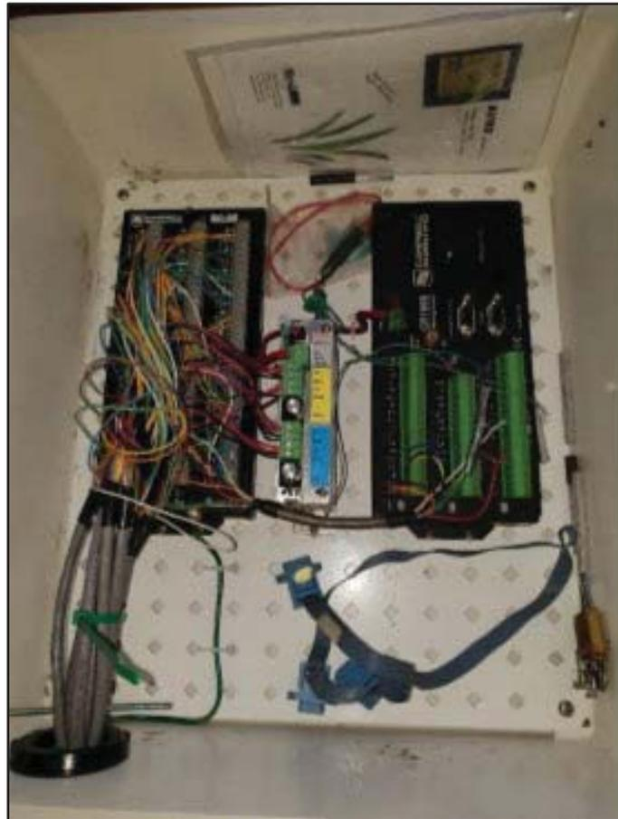
**Plate 4-11: The wiring of the Dynamax system with a CR1000 data logger and an AM16/32B multiplexer with two adjustment potentiometers of the adjustable voltage regulator in the centre**
