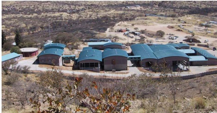
Figure C-3: The Goreangab Water Reclamation Plant (Wingoc, 2014)
