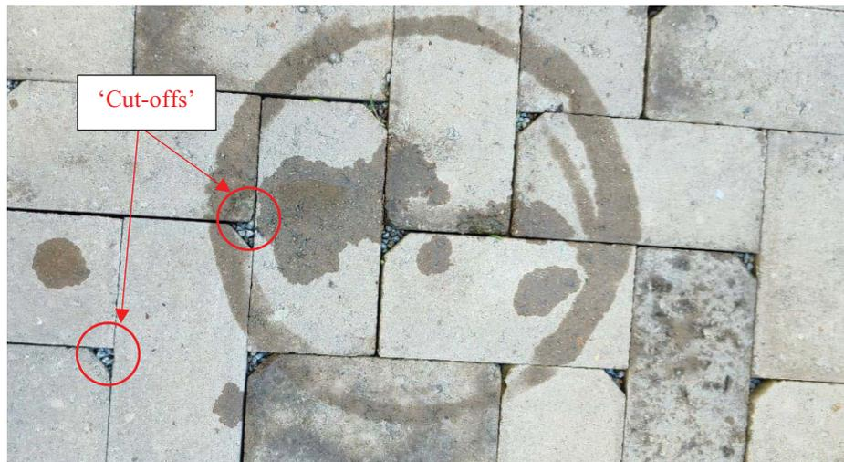
**Figure 4-92: Typical 'cut-off' pavers**
