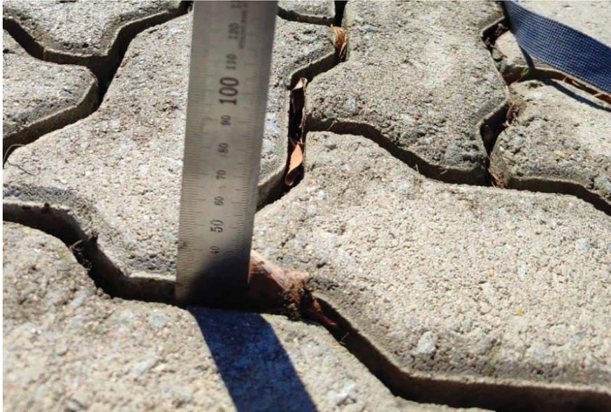
**Figure 4-66: BRT-7-03 missing gritstone (up to 30 mm)**
