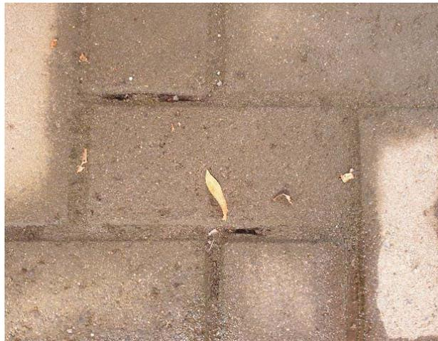
**Figure 4-74: Typical sediment accumulation in joints adjacent to vegetated areas**
