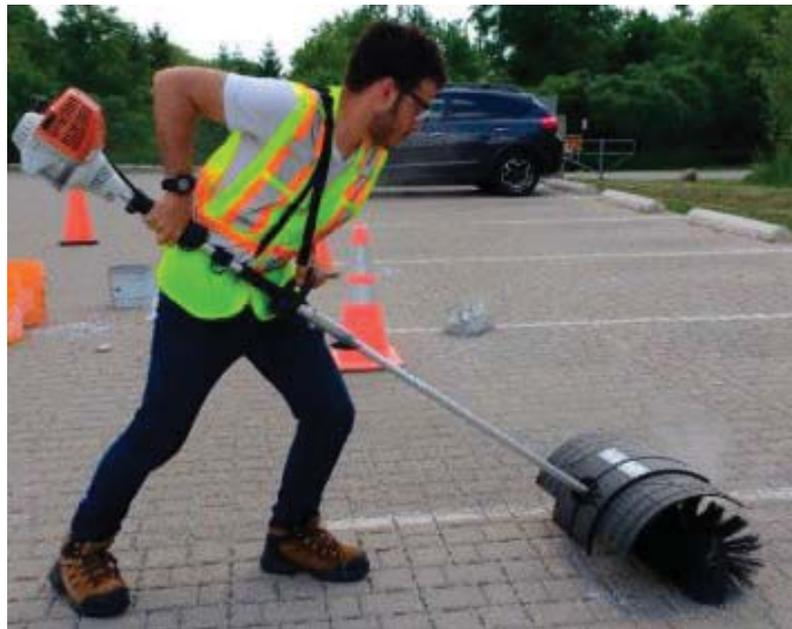
**Figure 2-32: Application of a power brush (Sehgal *et al.*, 2018)**
