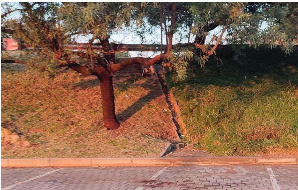
**Figure 4-101: Typical concrete-lined chute between WITS-U and WITS-L**
