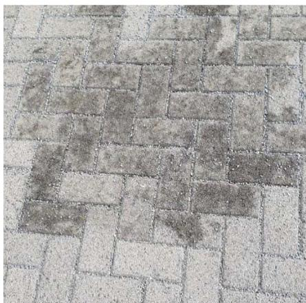
**Figure E-7: Repaired PICP test spot**
