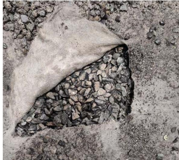
(b) Geotextile and choke layer
