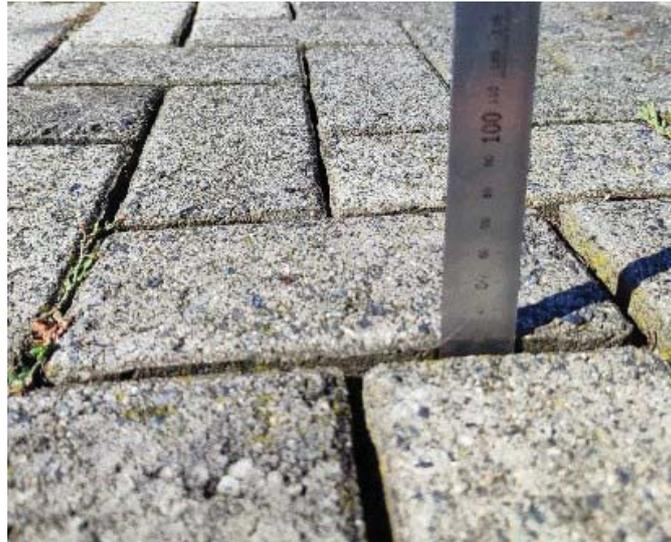
**Figure 4-85: Typical PICP section with missing grit**
