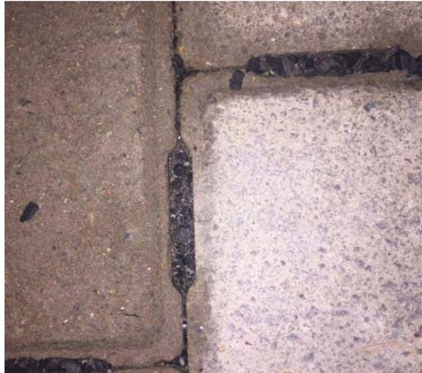
**Figure 5-15: Typical sediment accumulation between the Aquaflow<sup>®</sup> pavers**
