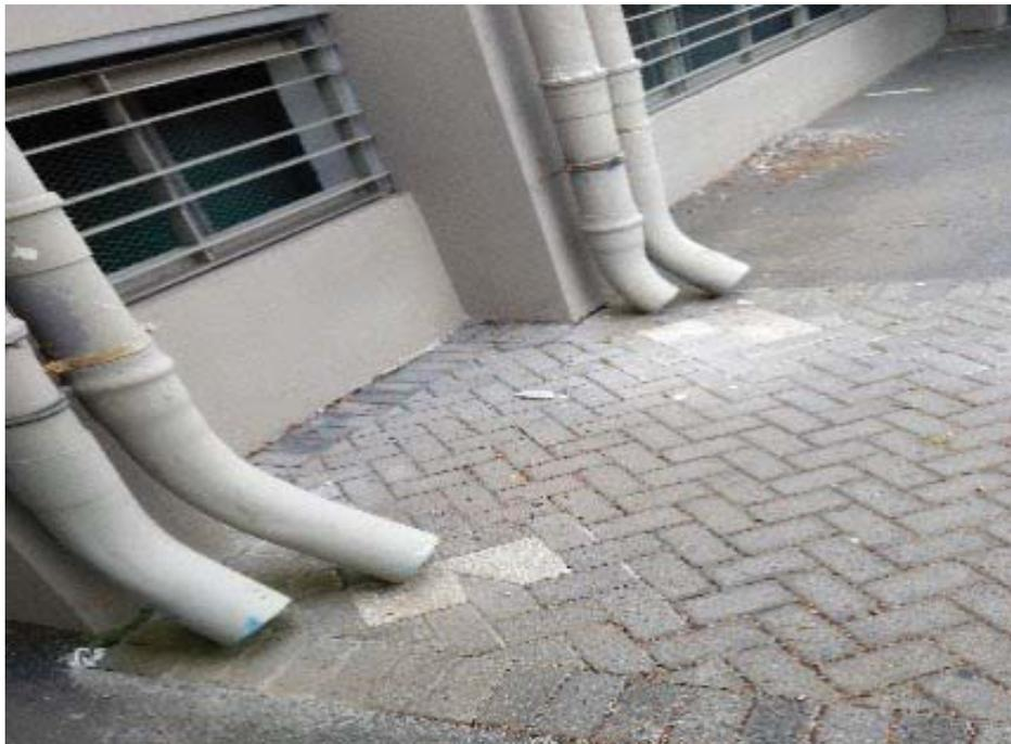
**Figure 4-7: Roof downpipes draining onto the PICP**
