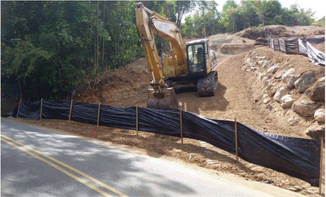
**Figure 2-20: Inadequate sediment trap installation** (St John Source, 2022)
