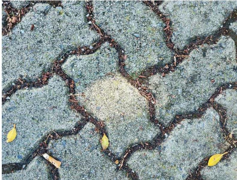
**Figure 4-64: Typical Area 2 sediment and organic filled joints**
