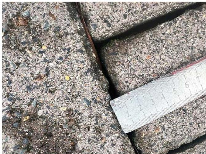
**Figure 4-25: Typical PICP section with missing grit and fine sediment on the pavers**
