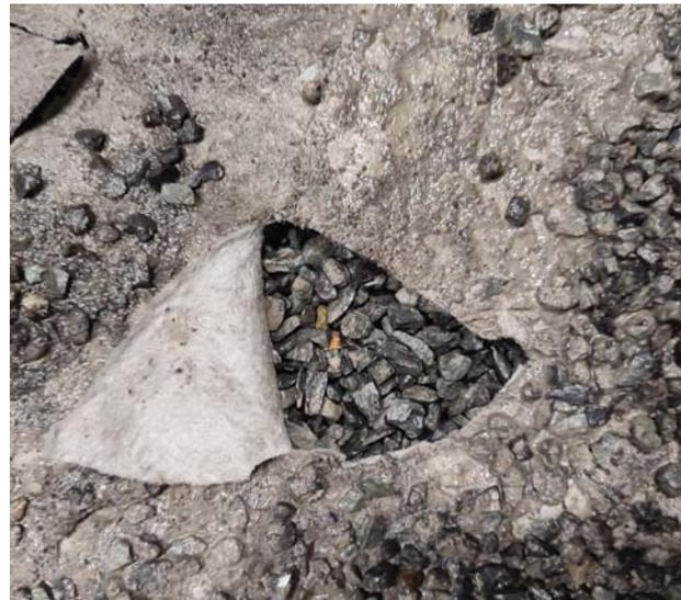
(b) Geotextile and choke layer
