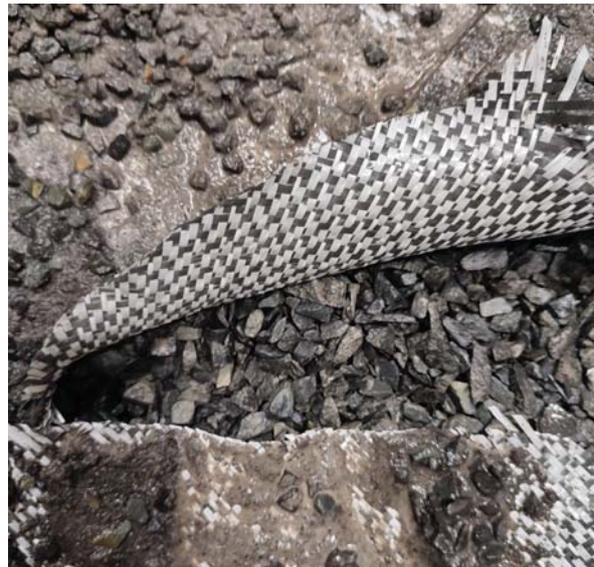
(b) Geotextile and choke layer
