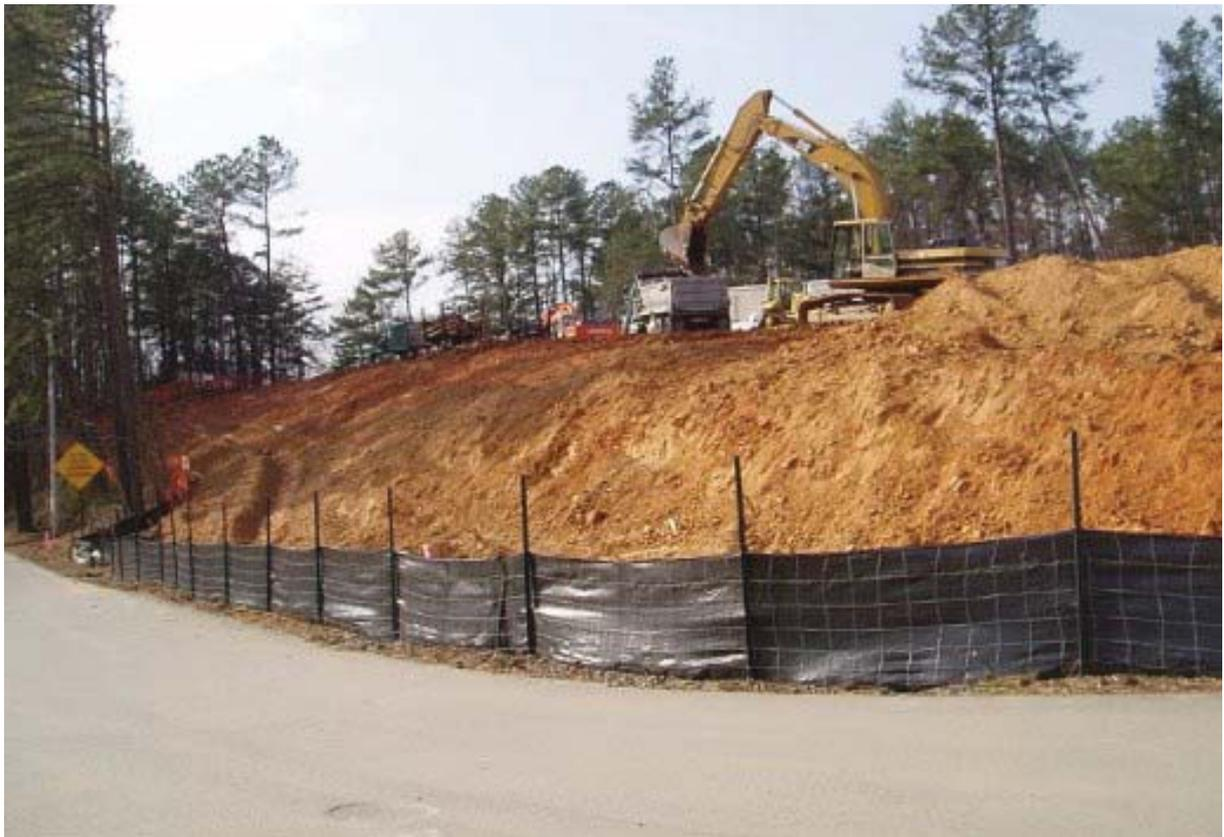
**Figure 2-19: Sediment trap** (Industrial Fabrics, 2022)
