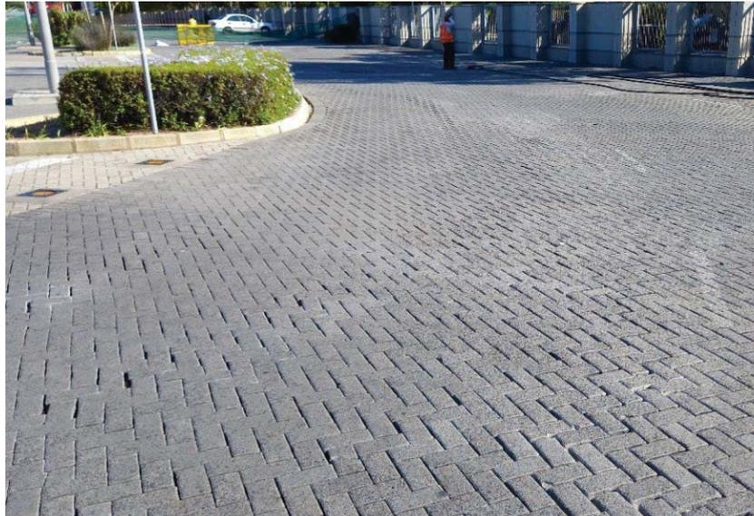
**Figure 6-8: A failed PICP edge restraint at a bend in the road**
