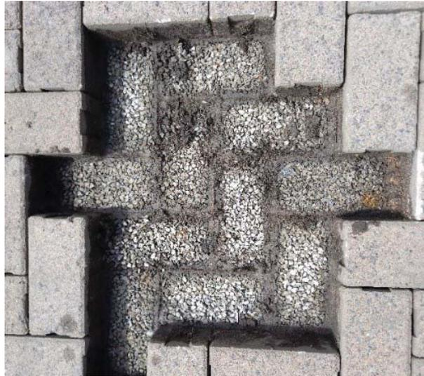
**Figure E-2: Type II clogging (below the joints)**
