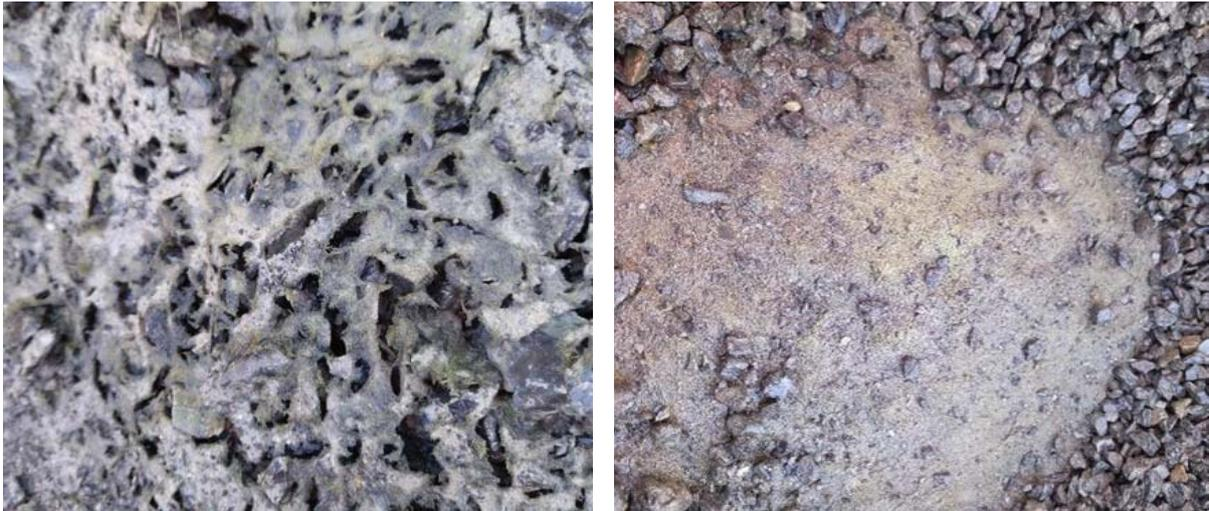
**Figure E-4: Top geotextile failure**
