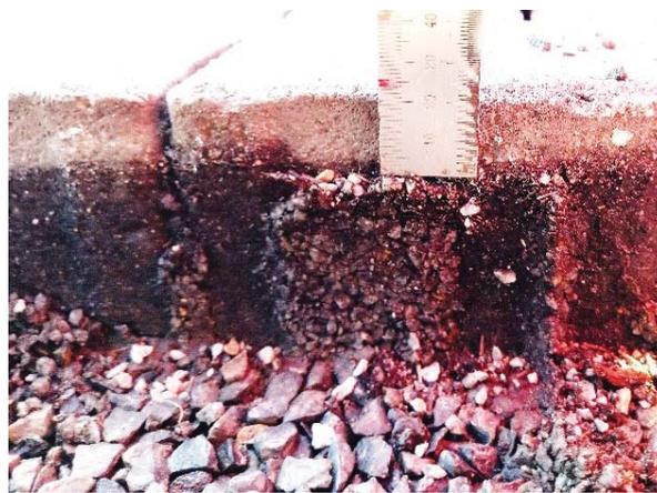
**Figure E-1: Type I clogging (in the joints)**
