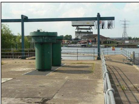
Measuring weirs provide an example where hydropower installations can be considered. The potential available at this type of location can be attributed to the large flow and elevation difference created by the weir. The challenge, however, would be to install a hydropower plant without affecting the accuracy of the measuring weir.
