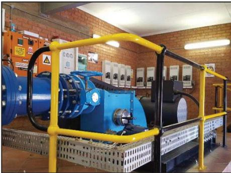
Pressure reducing stations (PRS) are constructed on gravity fed bulk water supply lines to dissipate excess pressures that might exist by means of a pressure reducing valve (PRV). The opportunity for energy recovery exists at the PRV, where the hydropower installation bypasses the PRV and uses the excess pressure for energy generation.
