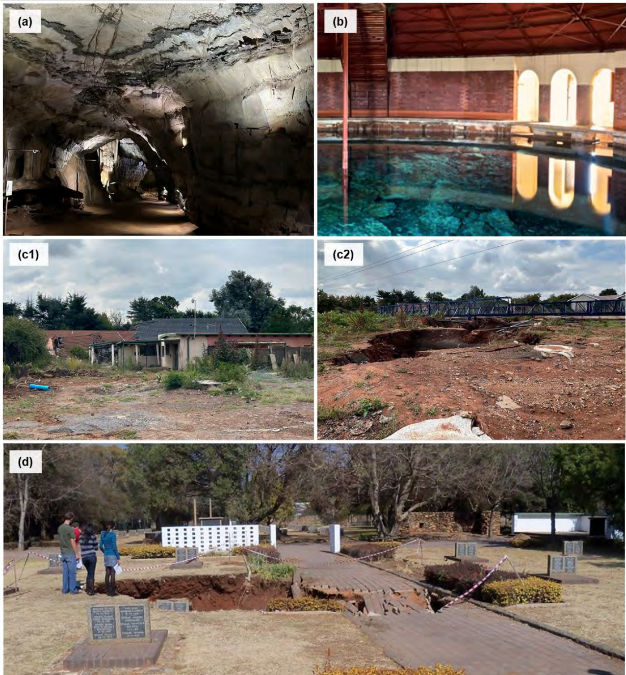
Figure 4-11 (a) Grootfontein spring providing Pretoria with drinking water (photograph by Gerrit Burger), (b) and (c) sinkhole falling due to leaking pipe and destroying houses; (d) sinkhole due to leaking irrigation pipe in cemetery (photographs by Dippenaar).
