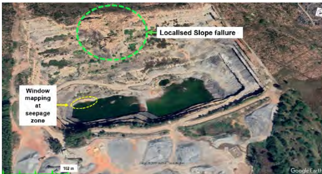
Figure 5-1 Google Earth image showing localised planar slope failure and geotechnical window mapping location in the quarry pit.
