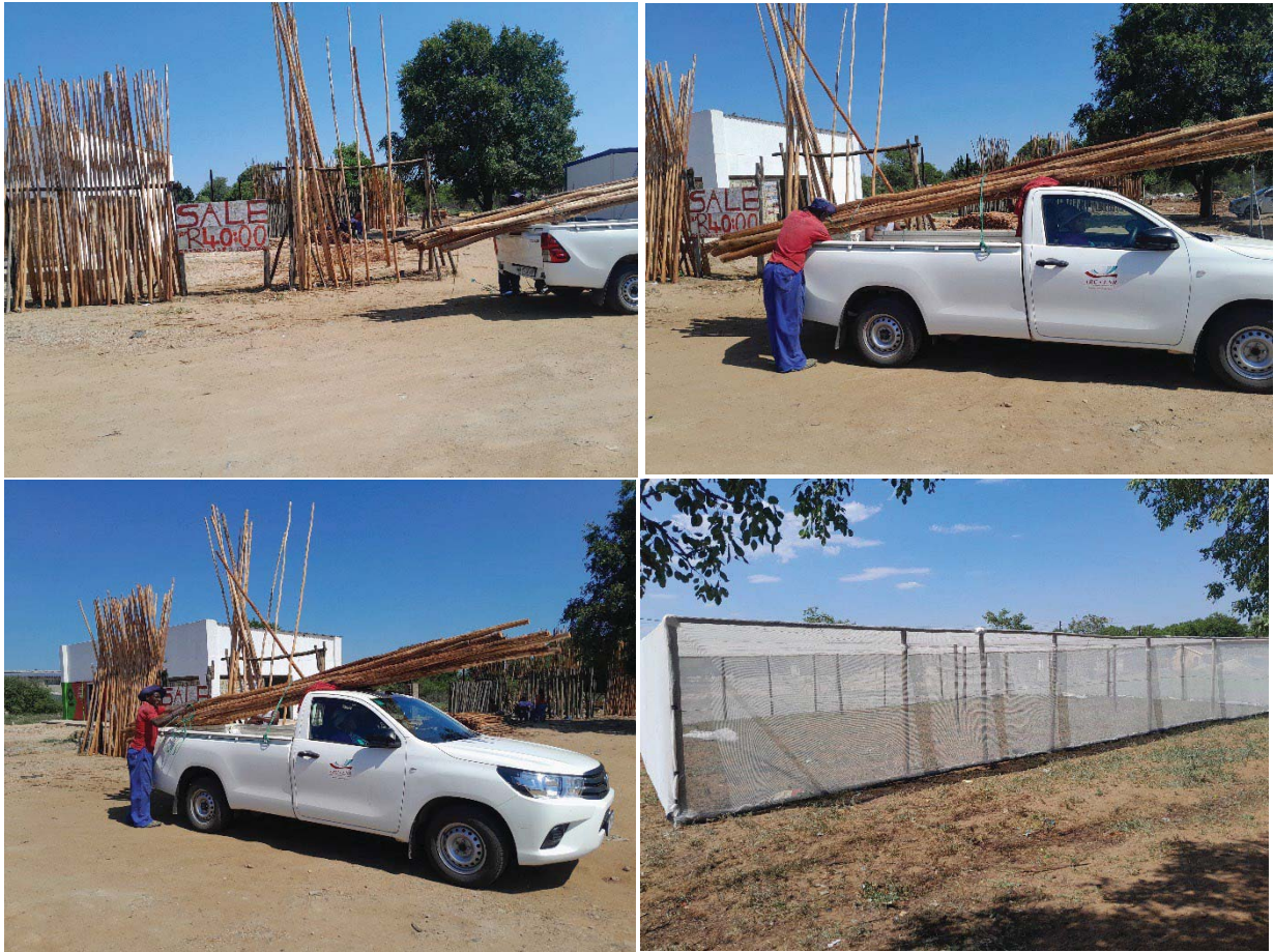
Figure 5-16: Wooden poles were sourced from local businesses to construct shade net structures at the co-operatives and schools.
