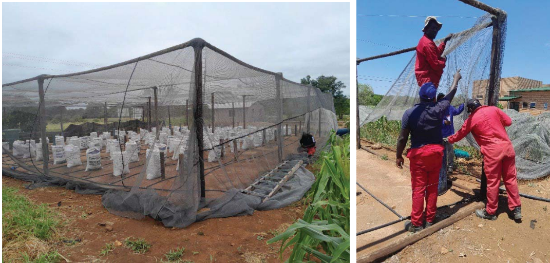
Figure 5-11: Renovated nursery at Muyexe Co-operative Project.
