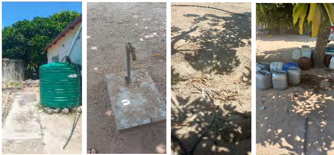
Figure 35: Left to right. A cement rainwater harvesting tank, installed by Mvula Trust, is no longer operational and replaced by a 2,2 kL Jo-Jo tank in a household in Turkey 2. And the old Mvula Trust tap is no longer operational. A small pipe from an individual borehole and collection containers for a group-based scheme.
