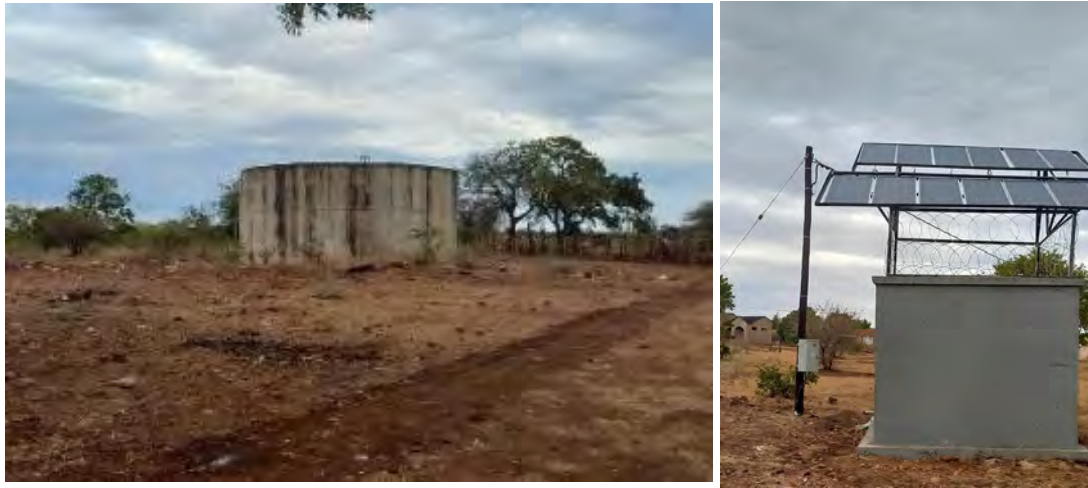
Figure 30: A view of the 700 kL village header tank in Mayephu and one of the boreholes supplying this tank fitted with electricity from both a power line and solar panels, for dual supply
