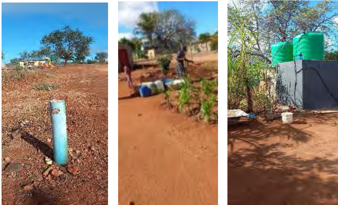
Figure 31: Water access options in Mayephu village: communal standpipes, yard connections with some storage, private boreholes with more substantial storage
