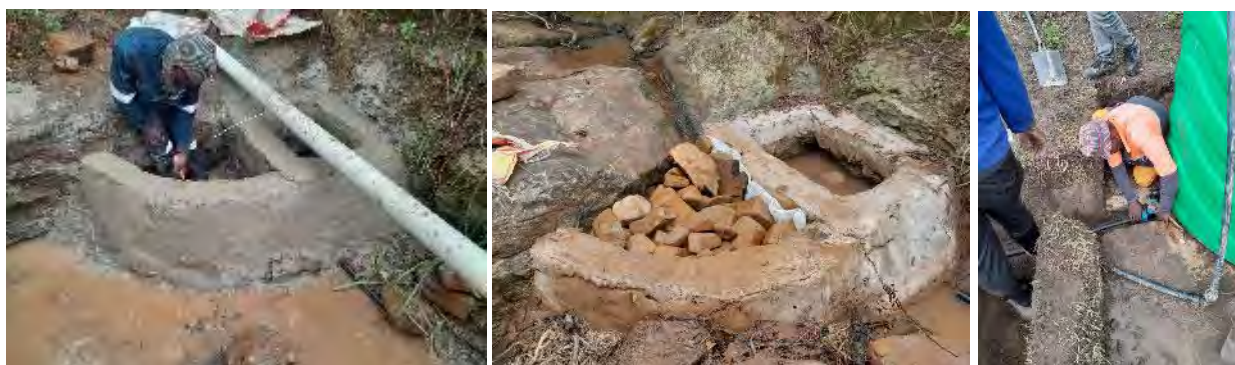
Figure 38: Left to right: Construction of the weir and v-box in the stream for both sections A and B. The finalised weir, with shade cloth and rocks in the inlet chamber and the brake pressure tank (92,5 kL) with pipes connected from the source and towards the header tank – also for both sections
