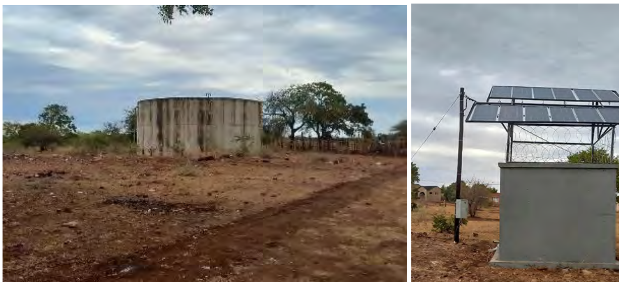
Figure 8: A view of the 700 kL village header tank in Mayephu and one of the boreholes supplying this tank fitted with electricity from both a power line and solar panels, for dual supply
