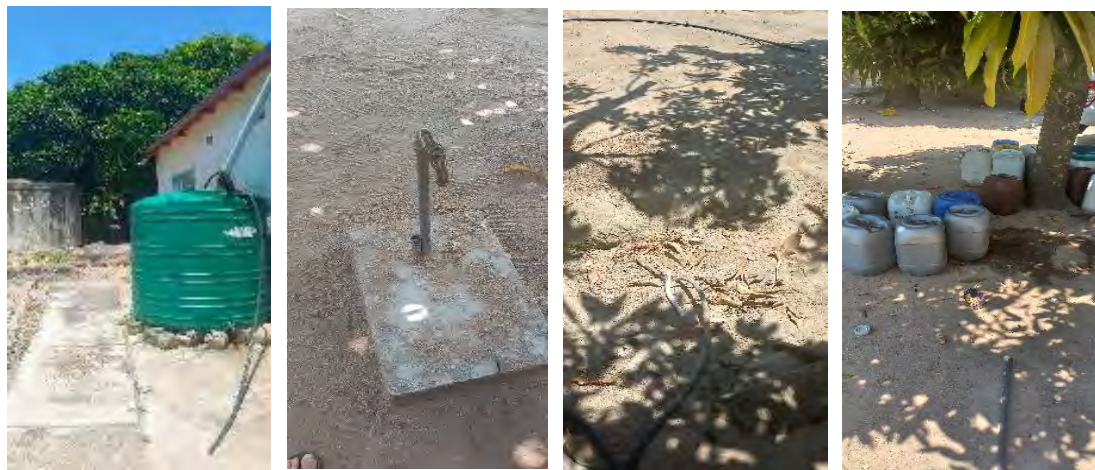
Figure 13: Left to right. A cement rainwater harvesting tank, installed by Mvula Trust, is no longer operational and replaced by a 2,2 kL Jo-Jo tank in a household in Turkey 2. And the old Mvula Trust tap is no longer operational. A small pipe from an individual borehole and collection containers for a group-based scheme.
