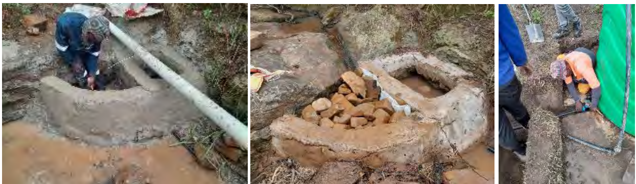
Figure 19: Left to right: Construction of the weir and v-box in the stream for both sections A and B. The finalised weir, with shade cloth and rocks in the inlet chamber and the brake pressure tank (92,5 kL) with pipes connected from the source and towards the header tank – also for both sections A and B
