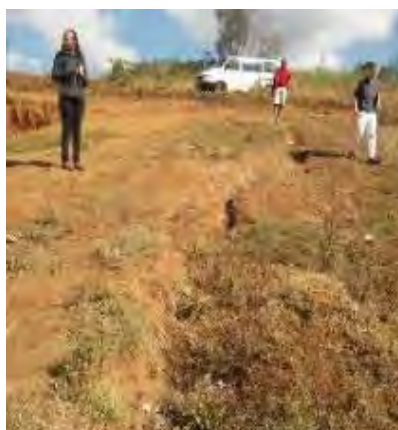
Gully forming in a field
