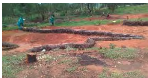
Above: Pictures showing the smoothing of the bank edges, then the lines of pegs placed on contour and filled with brush from cleared wattle. The picture on the bottom right shows a brush pack after a period of time with siltation starting on the upslope of these packs.
