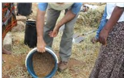
Both the gravel and sand is rinsed prior to use, to make sure they are clean and to avoid clogging up of the system (2015)
