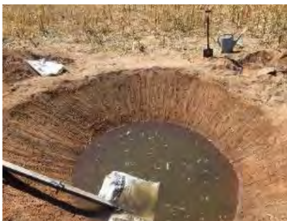
A small pond lined with bentonite (the yellowish clay inside the pond,) being filled up. Note the angle of the pond walls, the slope of the pond walls, that allows for the bentonite to be stamped into sides and bottom of the pond to seal it.
