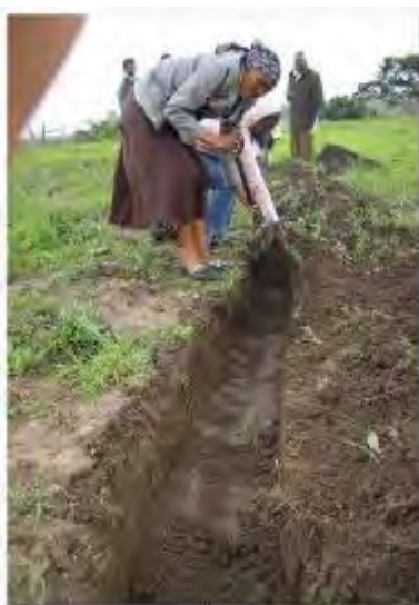
Digging the cut off drain/swale ditch. Soil is placed on the downslope
