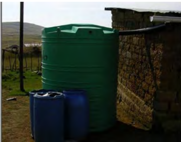
Gutters and inlet pipes are important when using Jo-Jo tanks to collect water from roofs
