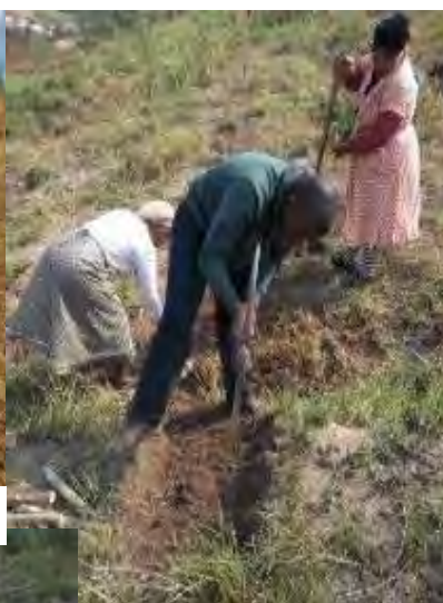
Digging the ditch for keying in the stones for the check dam
