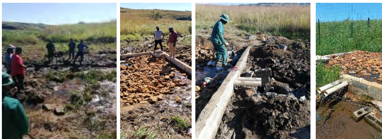
Above Left to Right: The original spring before protection in Stulwane, Bergville. The catchment wall has a V-box in the bottom corner and is covered with rocks, gravel, and sand towards the eye. Building in the overflow pipes. The protected spring has a fence around it to protect it and a small catchment area above the spring.
