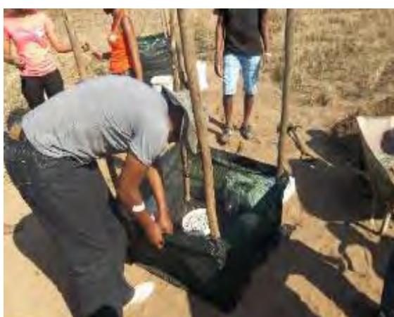
Placement of the stone column – in the small bottomless bucket in the middle of the bed
