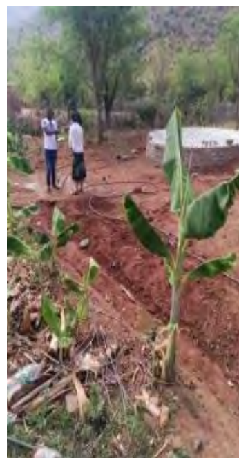
A completed geofabric tank with brick wall and roof for safety. The inlet furrow for water is in the foreground
