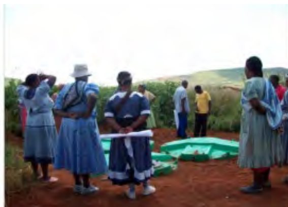
Jo-Jo tanks buried for underground water storage
