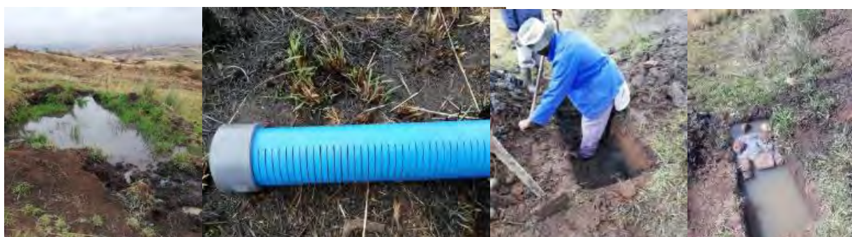
A spring dug out to form a small dam. The spring protection consists of a slotted pipe buried in a ditch dug below the dam and which is then covered with gravel, shade netting and soil, to be protected. In this way a spring can be protected, without major
