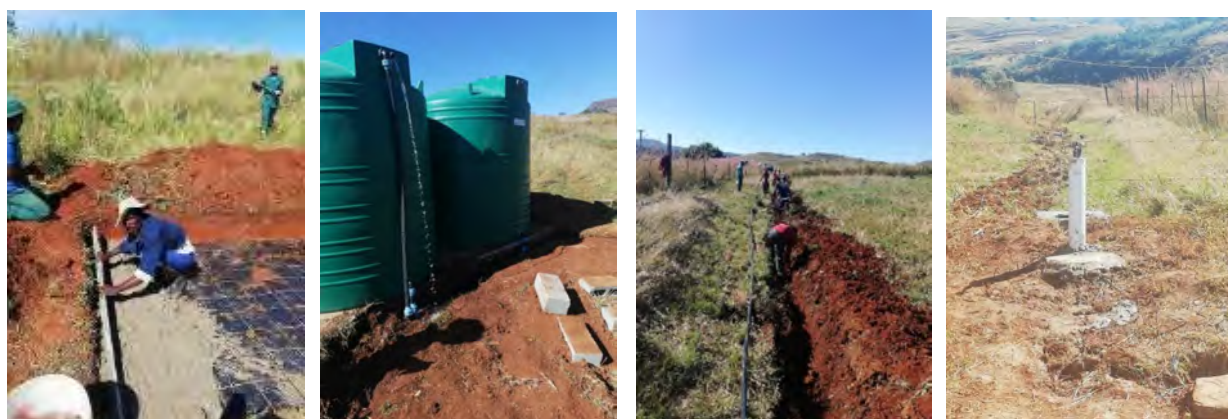
Above Left to right: Construction of the cement platform for the tanks. The two joined 2500l JoJo tanks. Digging ditches and laying pipes for the community taps. An example of a community tap upon completion.
