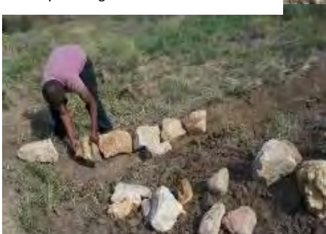
Starting to pack the check dam. Large rocks go at the bottom
