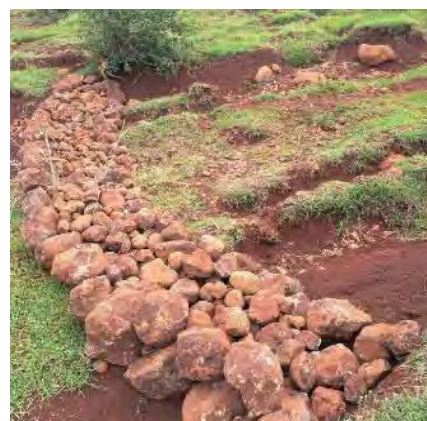
The two pictures above show different variants of stone lines used across slopes with multiple small channels, which are developing into a gully/donga.
