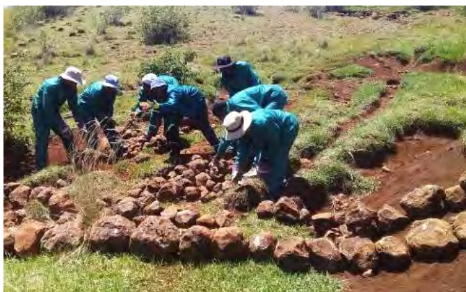
The two pictures above show different variants of stone lines used across slopes with multiple small channels, which are developing into a gully/donga.
