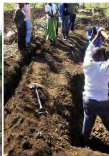
Preparing trench beds below a swale
