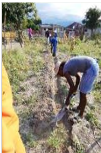
Digging out a shallow trench 30cm wide and 15cm deep on a contour line in a field
