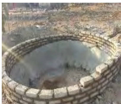
A ferrocement underground tank with brick wall for placement of a roof structure under construction
