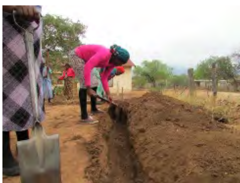
Digging a diversion ditch (1,5-5% slope; 30cm wide and 30cm deep) with soil placed on upper slope
