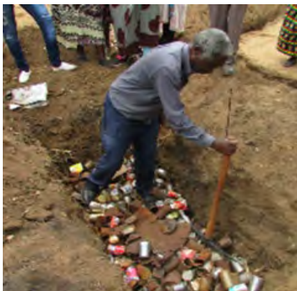
Imisele yembiwa ukusukela kuwashumi asithandathu ukuya kwimitha enye ukubanzi . Trenches are dug 60cm-1m deep. Umeleko ongaphantsi wenziwe ngeetoti ezindala okanye branches
