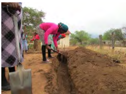
Ukugrumba umselele ophambukisa amanzi (kwithambeka elifika kwisihlanu ukwenyukela, kube ngamatshumi amathathu ububanzi, kwaye namatshumi amathathu ububanzi, ube umhlaba ubekelwa ngasenhla kwithambeka
