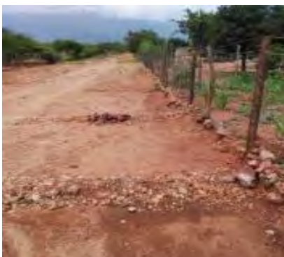
Amatshe amancane asebenzisela okulwawula ukugeleza kwamanzi emgwaqeni awahambise ezingadini
