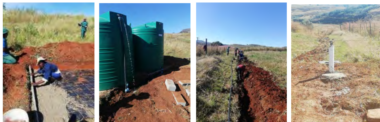
Ngenhla kusuka kwesokunxele kuya kwesokudla: ukwakhelwa kwamathangi indawo yokuhlala ngo simende. Amathangi amabili ayizi-2500 wamalitha axhumene, ukumbiwa kwemisele nokufakwa kwamapayipi aya kompomp. Isibonelo sompomp womphakathi uma sekuqediwe.
