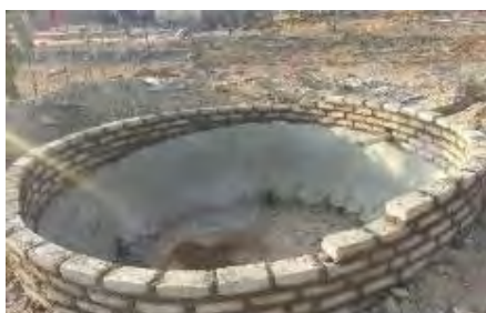
Ilthangi leferrocement eligujelwe ngaohansi elinodonga lwezitini ukwakhela indawo yokubamba amanzi nophandla nslusakhiwa
