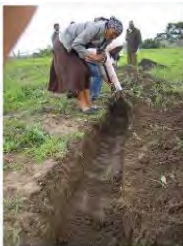
Ukumbiwa kwe -swale inhlabathi ibekwa ngasohlangothir olwehlelavo
