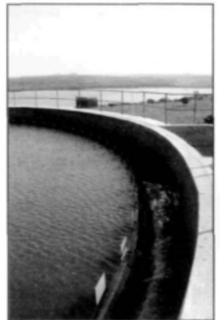
Figure 9: Photograph of sedimentation unit
