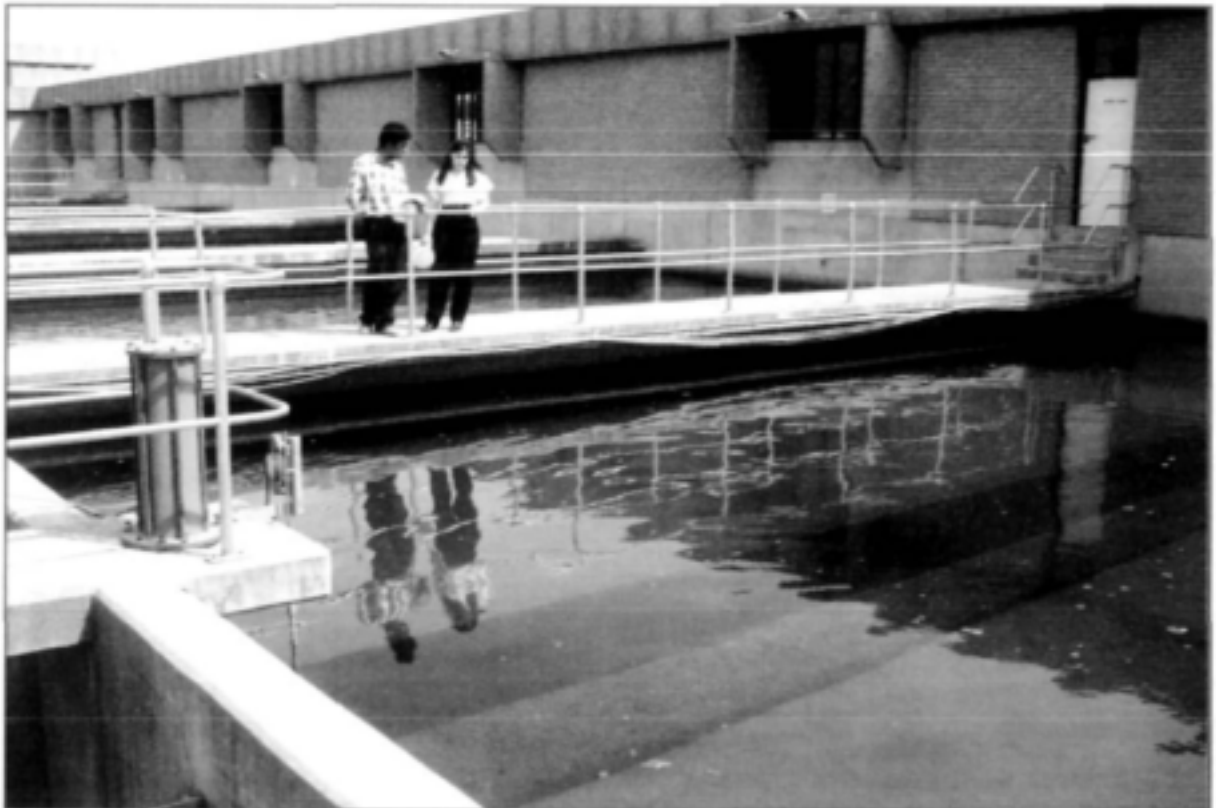
Figure 12: Photograph of rapid gravity sand filter
