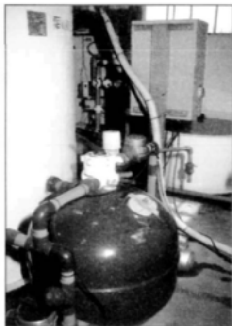
Figure 13: Small-scale pressure sand filter
