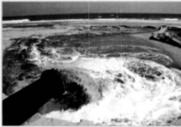
Dredged spoil being discharged onto the beach at St Lucia (Picture: Ricky Taylor)
