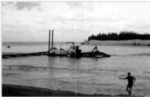
Dredger at the mouth of the St Lucia Estuary (Picture: Bruce Mann)
