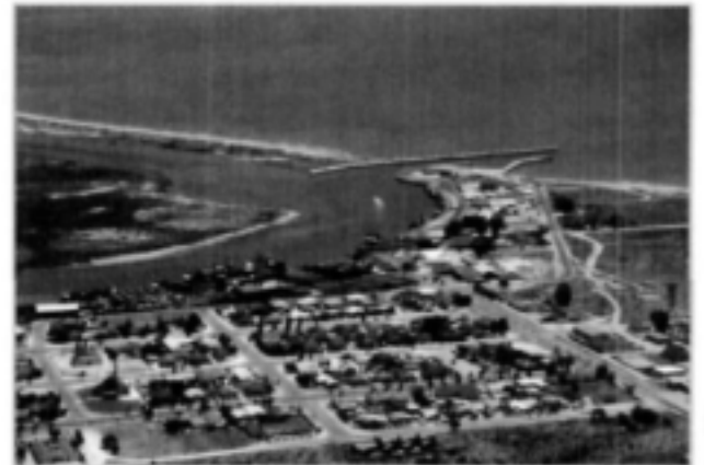
The breakwater at Laaiplek Estuary (Picture: CSIR)
