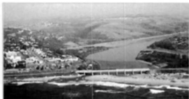
A train bridge built across the mouth of the Mkomazi Estuary (Picture: Dirk van Driel)
