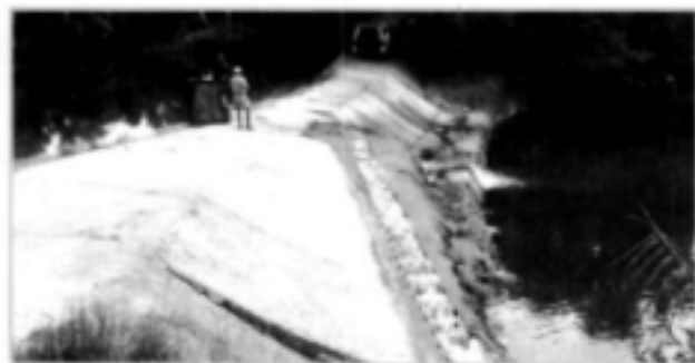
The weir at the head of the Kowie Estuary has a fish ladder to enable fish to migrate upstream (Picture: Anton Bok)
