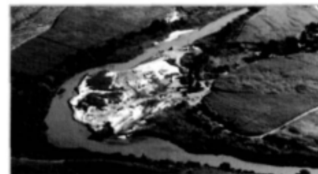
Sand deposited in the upper reaches of the Mdloti Estuary is removed for construction (Picture: Kevin Weerts)
