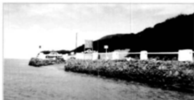
A bulkhead built on the bank of the Kariaga Estuary to provide parking (Picture: Margaret McKenzie)
